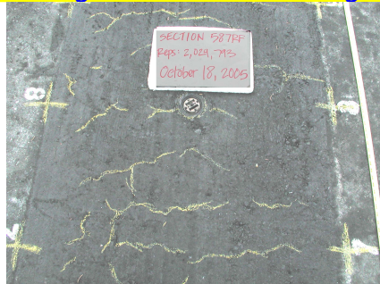
Cracking section after trafficking
