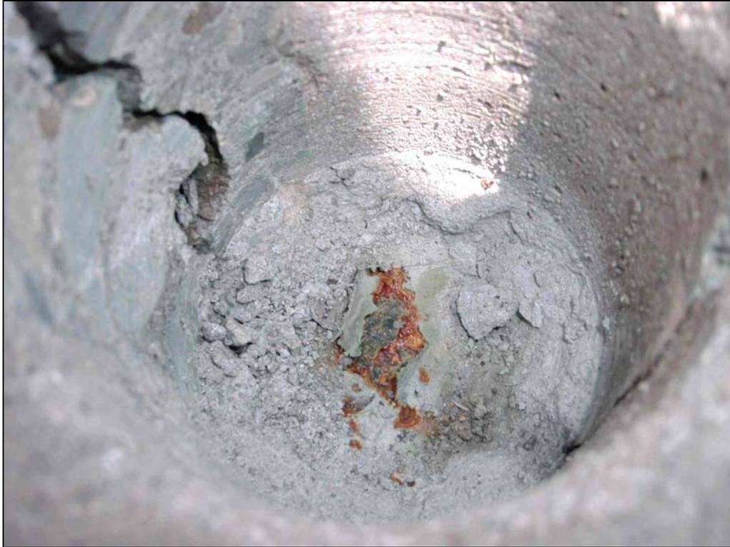
**Figure 55. View of the interior of a recently made core hole showing corrosion products underneath the epoxy coating.**
