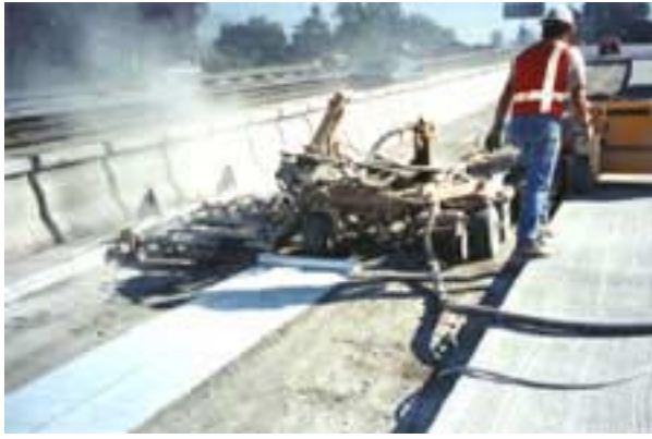
Figure 36. Self-propelled gang drill unit for drilling the bar holes to the existing slab.
