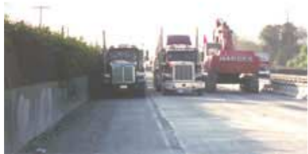
Figure 25. Excavator pausing operation to allow an end dump from other demolition team to pass.
