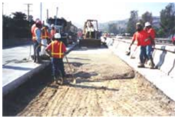
Figure 31. Placement of FSHCC CTB.
