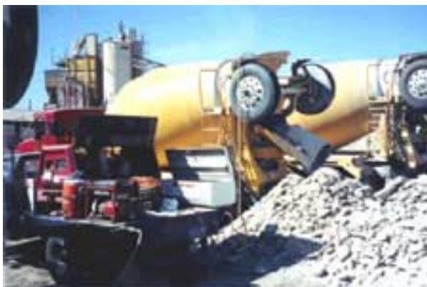
Figure 46. Chipping area at the batch plant.
