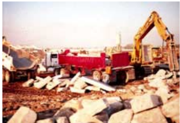
Figure 26. View of the dumping area with end dump trucks and breaker for rubblization.
