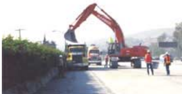
Figure 24. Concrete mixer truck waiting for clearance to pass behind the demolition operation.
