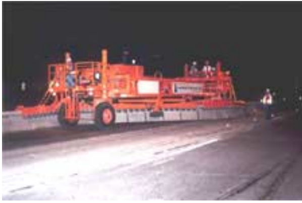
Figure 19. Installation MCB using transfer and transport machine.
