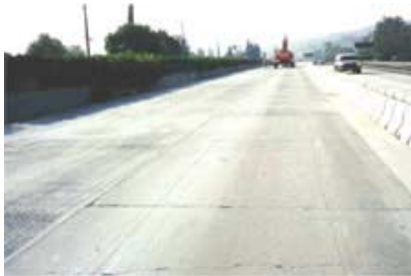
Figure 21. Slab panels cut into three pieces longitudinally.
