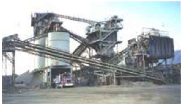
Figure 43. Vulcan Materials crusher plant (aggregate source).
