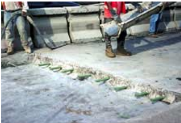
Figure 41. Placement of dowel bars in existing slab.
