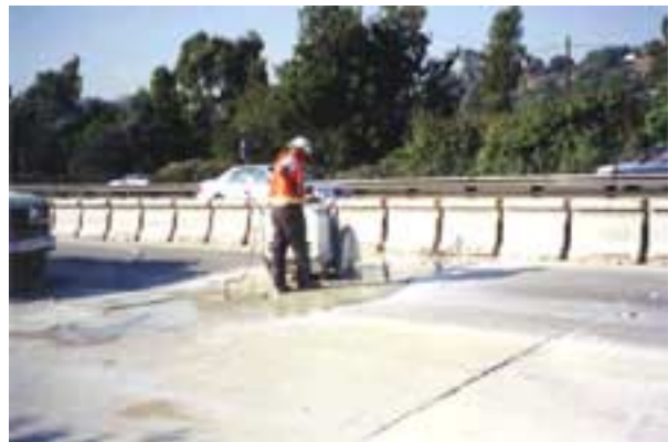
Figure 20. Slab cutting for non-impact demolition method.
