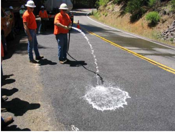
Figure 5. Application of water to patched area.
