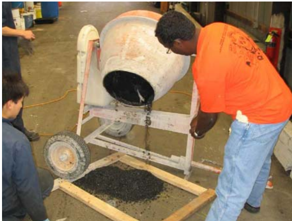
Figure 1. Patch material being placed in wooden frame on top of DGAC pavement.
