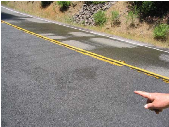
Figure 6. Water draining from downslope side of patched area.
