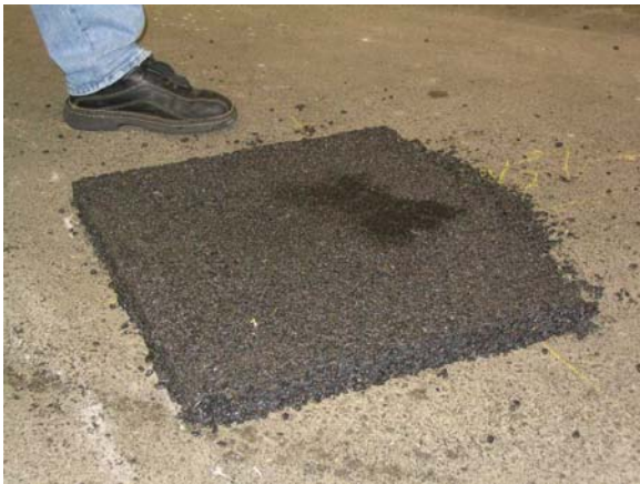
Figure 2. Water on surface of patch material.
