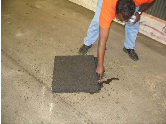
Figure 3. Water draining from downslope side of patch material.
