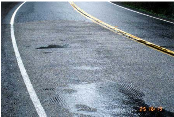
Figure 7. Deteriorated patch site showing significant raveling and roughness after one year.
