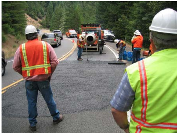
Figure 4. Placement of patch material on Highway 20 field site.
