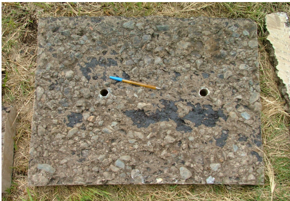
Investigation of slab underside
