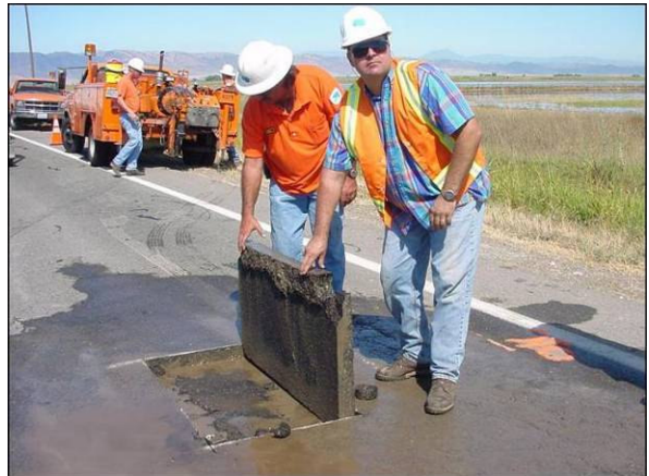
Slab removal
