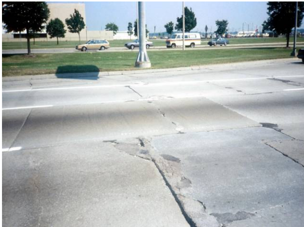
Inconsistent spalling, cracking, and faulting
