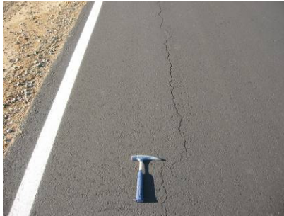
Longitudinal crack in new overlay
