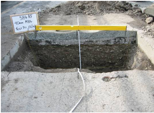
Total view of test pit
