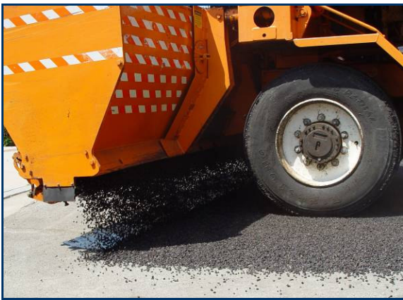
Chip spreader calibration
