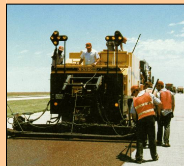
Microsurfacing application
