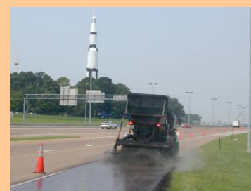
Shoulder fog seal
