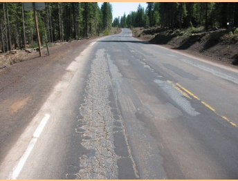
Inconsistent rutting and cracking
