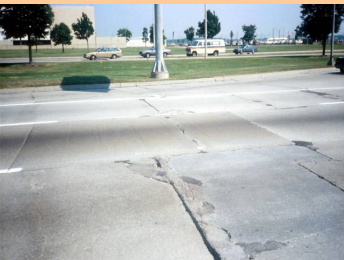
Inconsistent concrete surface
