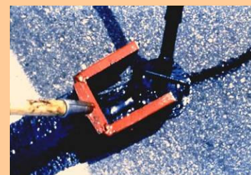
Crack seal
