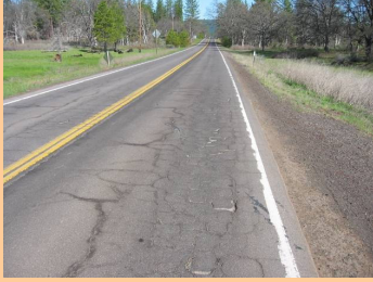
Consistent cracking
