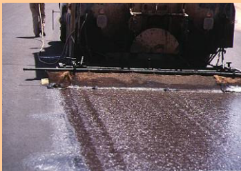
Slurry sealing
