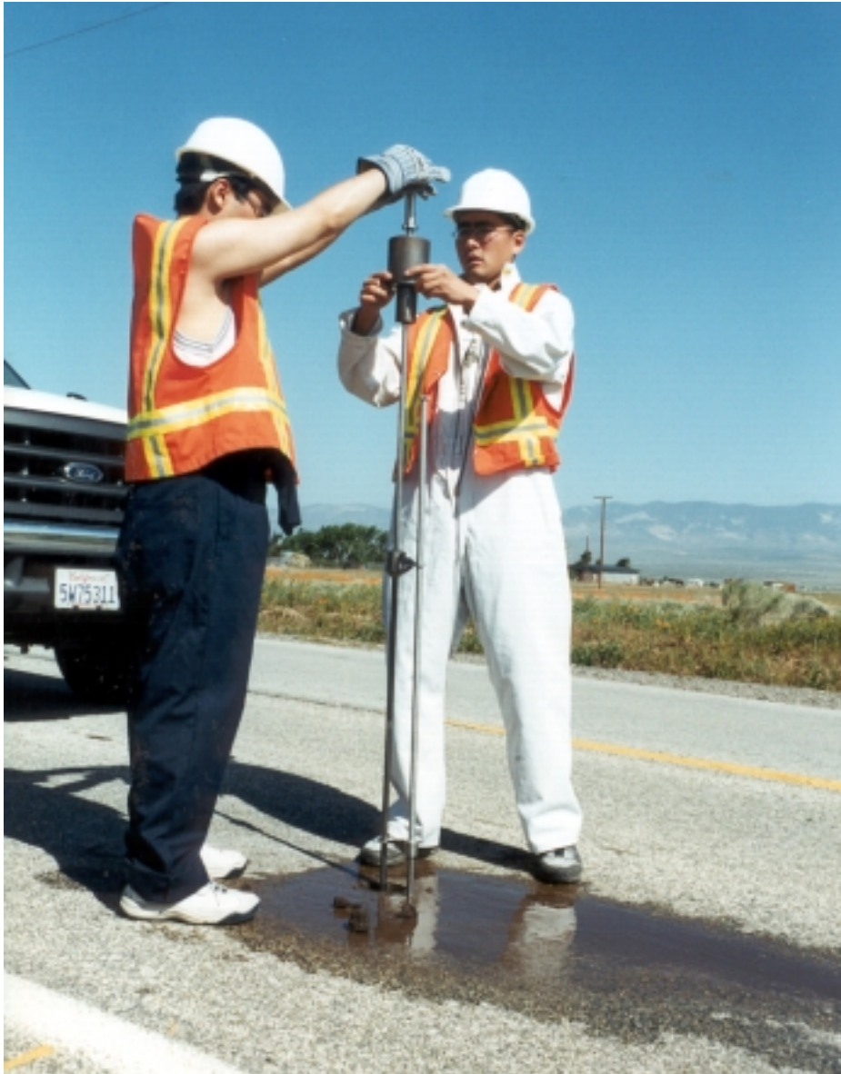
Figure 4. Crew performing DCP measurements on State Route 138.
