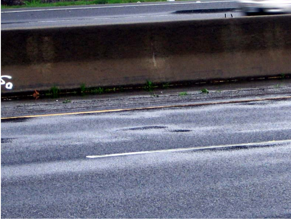
Figure 11. Ponding at Station 51+60 (inside lanes, southbound).
