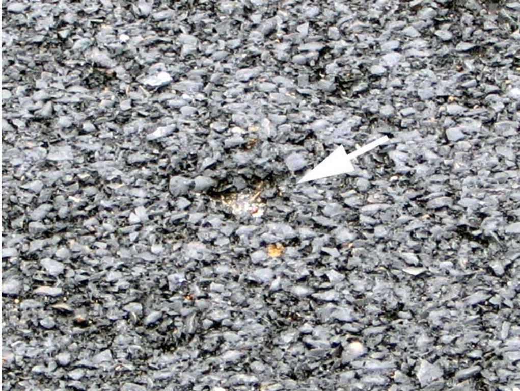
Figure 23. Hole at Station 56+80 (northbound direction).
