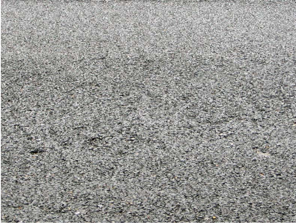
Figure 24. Raveling at Station 56+80 (northbound direction).
