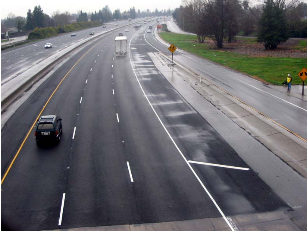
Figure 18. Ponding starting at Station 50+00 (outside lanes, northbound).
