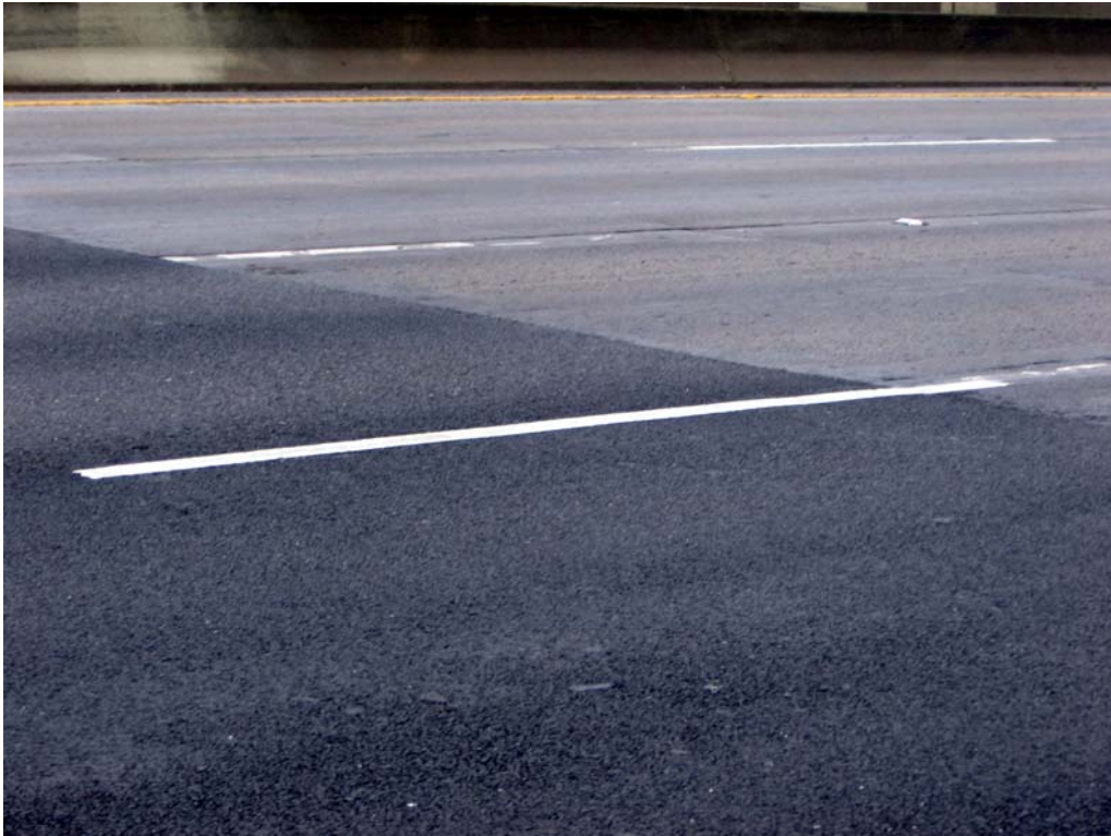
Figure 25. End of open graded section (northbound direction)
