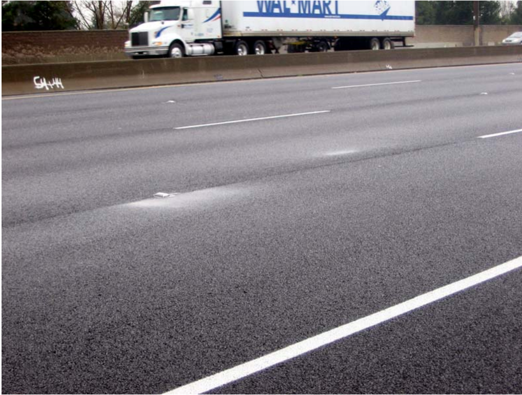
Figure 20. Ponding between at Station 54+44 (inside lanes, northbound).
