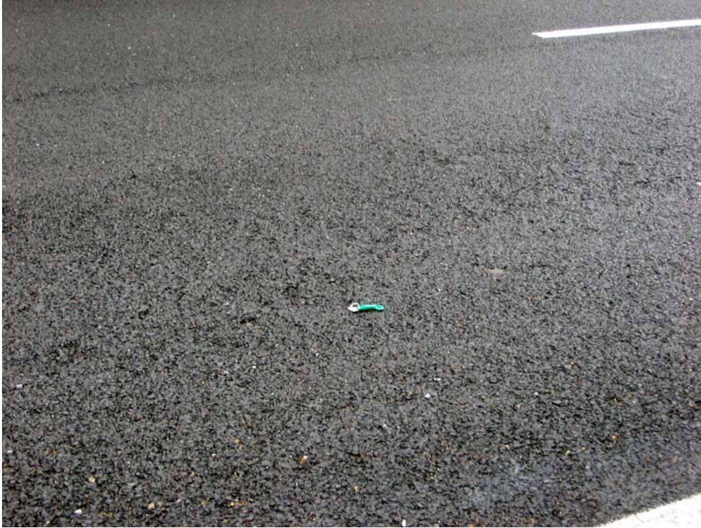
Figure 22. Raveling at Station 56+80 (northbound direction).
