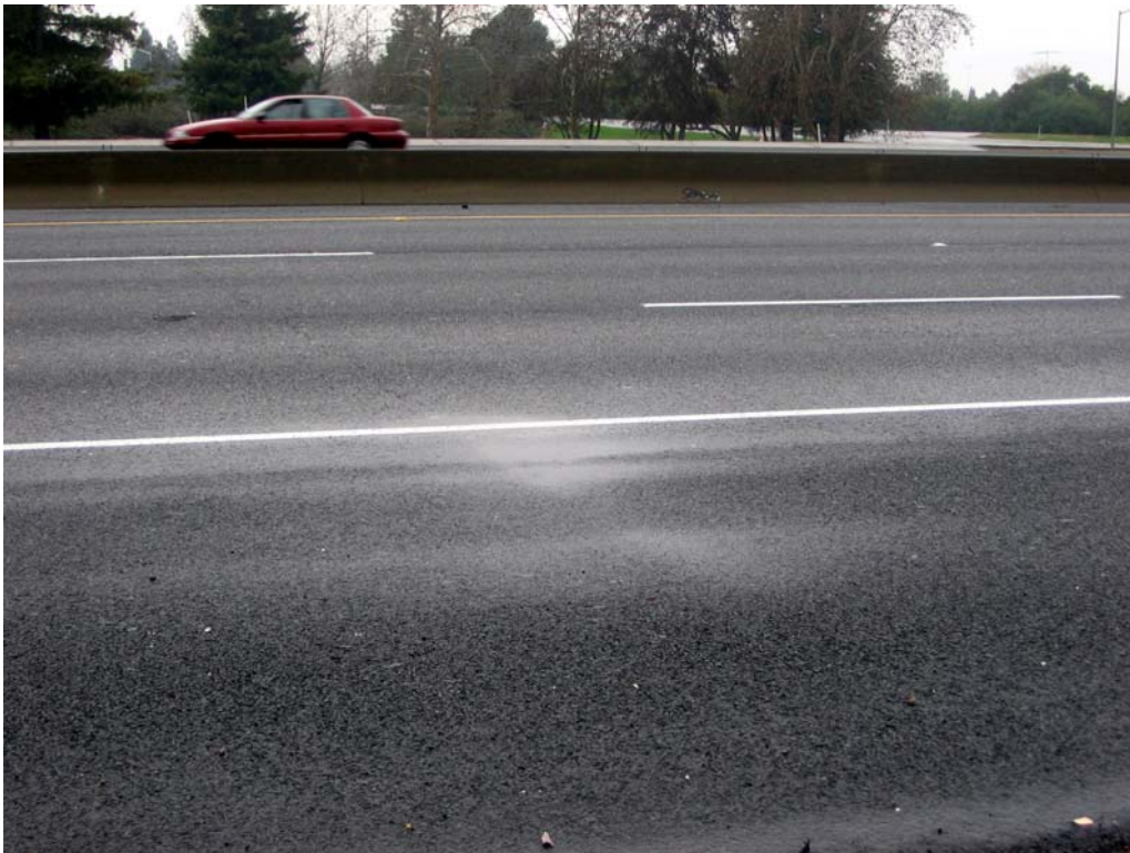
Figure 14. Reflection cracking between Station 51+00 and 52+00 (northbound lanes).
