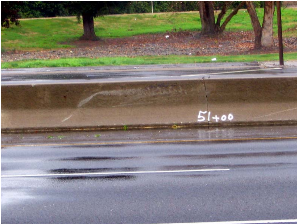
Figure 8. Ponding at Station 51+00 (inside lanes, southbound).
