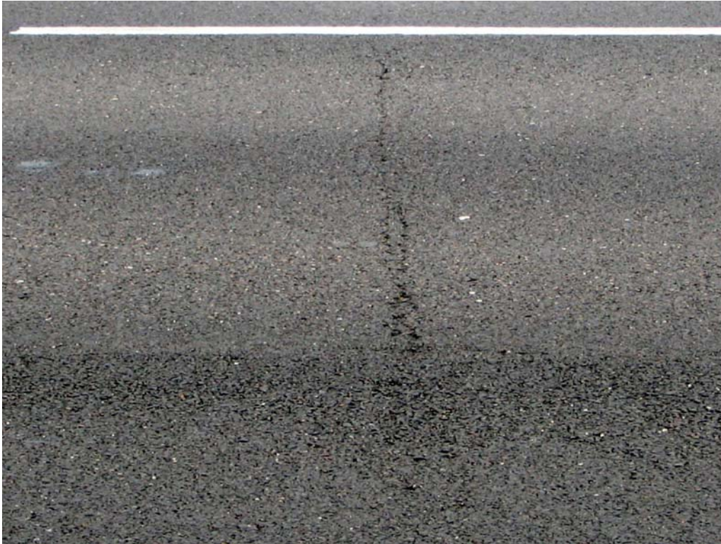
Figure 5. Reflection cracking between Station 51+00 and Station 52+00(southbound lanes).
