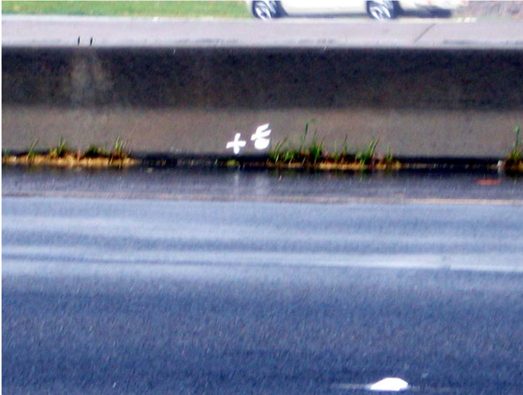
Figure 7 . Ponding at Station 50+40 (inside lanes, southbound).
