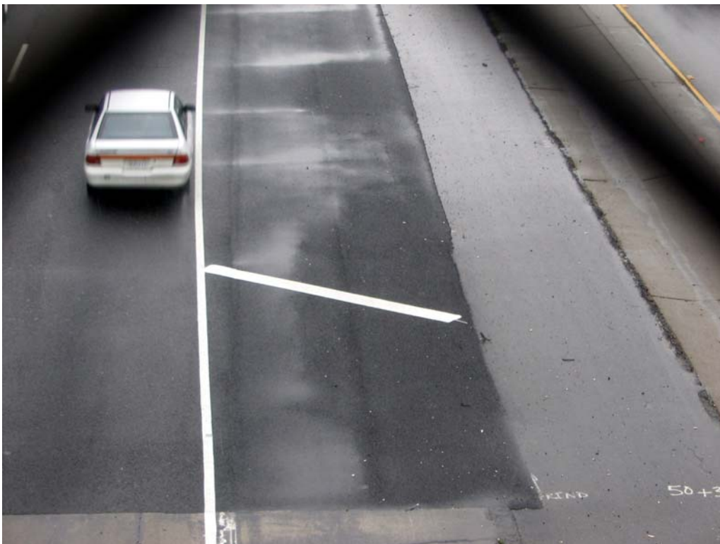
Figure 17. Ponding at Station 50+00 (outside lanes, northbound).
