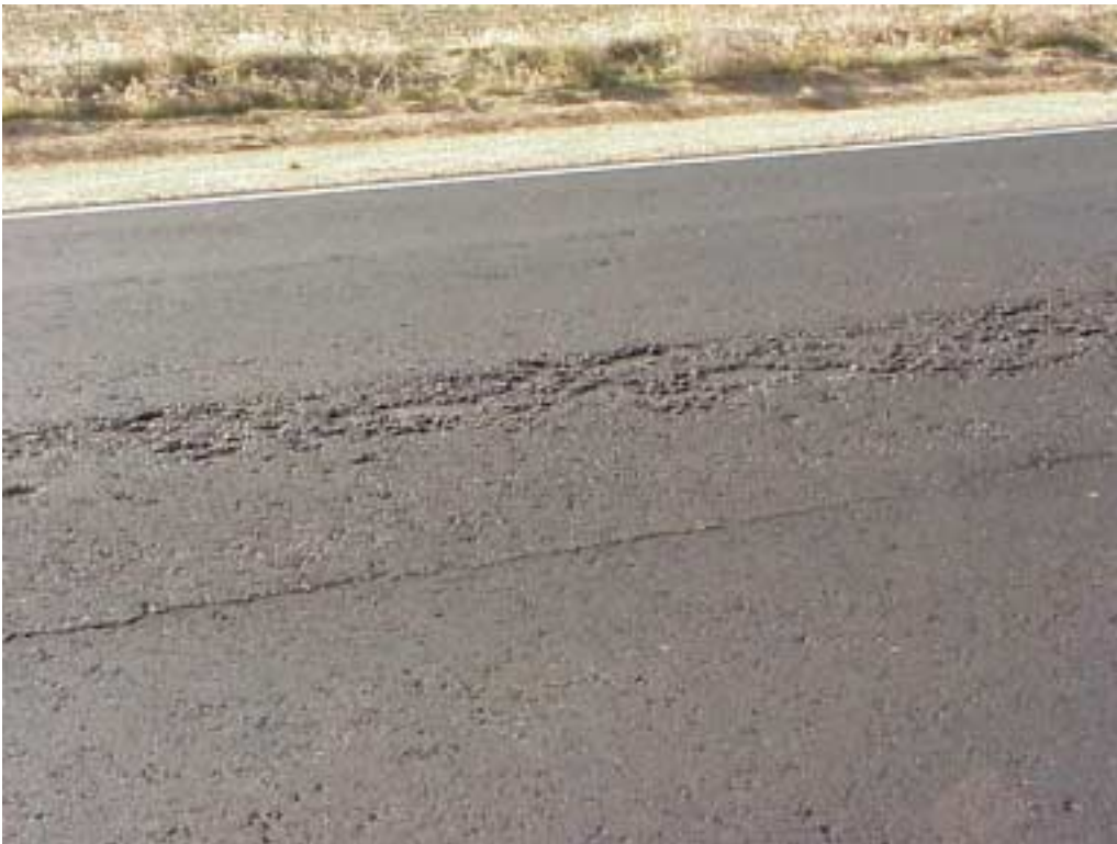
Figure B4. Area of segregation in levelling up course DGAC.
