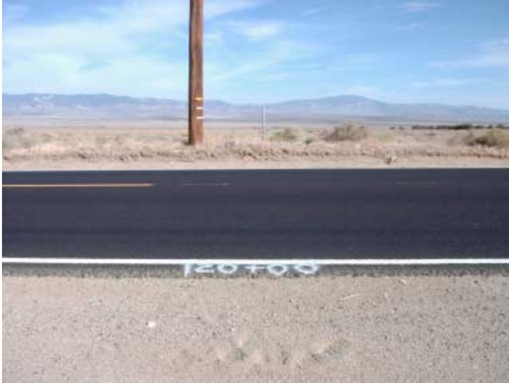
Figure D3. Transverse view of pavement at station 120+00 (30 mm OGAC).
