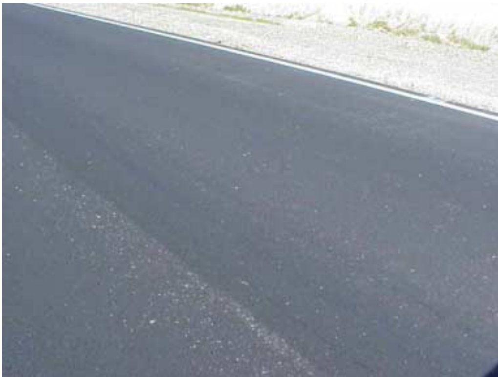
Figure B6. Area of segregation showing high and low oil contents in levelling course DGAC.
