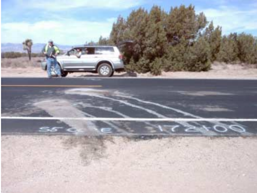
Figure D17. Transverse view of eastbound lane at station 172+00 (30 mm BWC), showing locations of cores.
