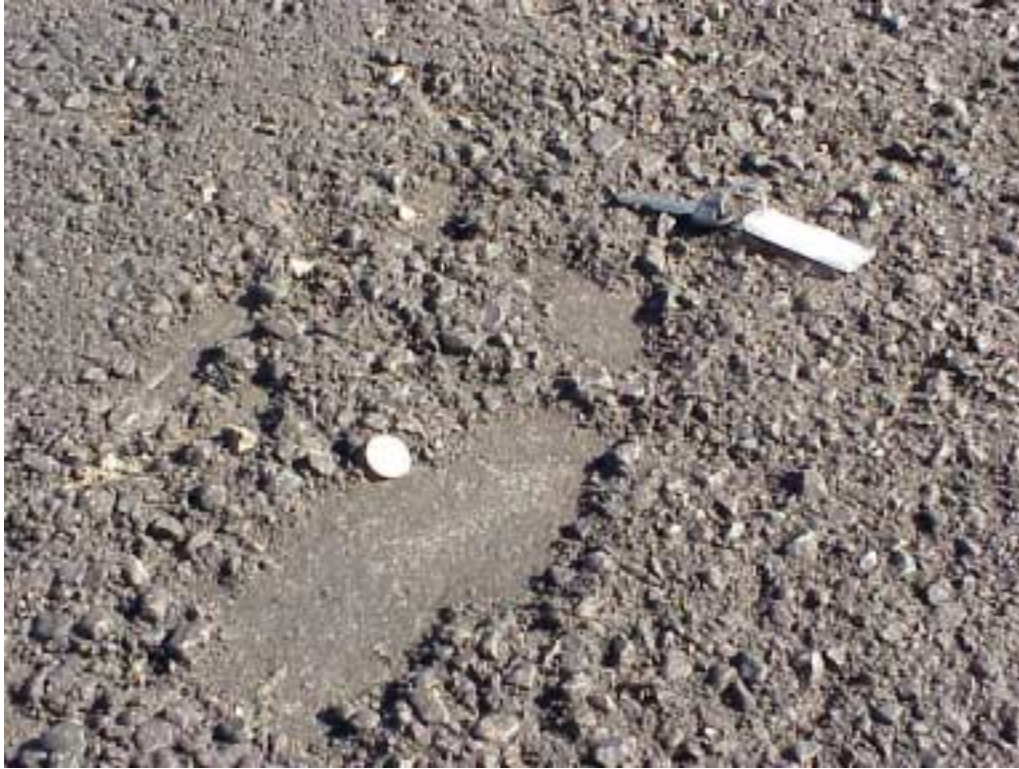
Figure B5. Close-up of segregated and ravelled area in levelling course DGAC.
