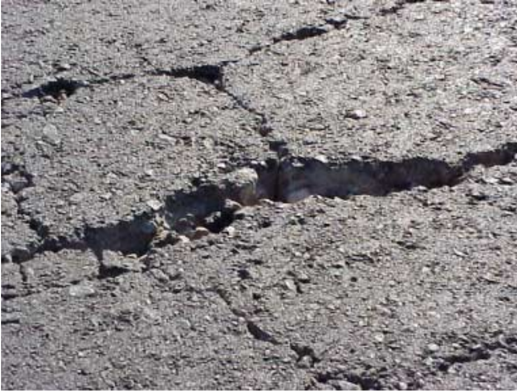
Figure B3. Close-up of localized reflection cracking showing thickness of DGAC layer.
