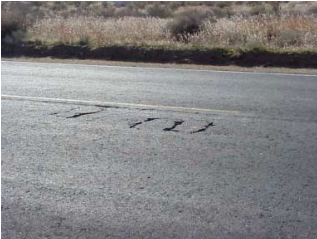
Figure B2. Area of localized reflection of wheelpath fatigue cracks through levelling course overlay.
