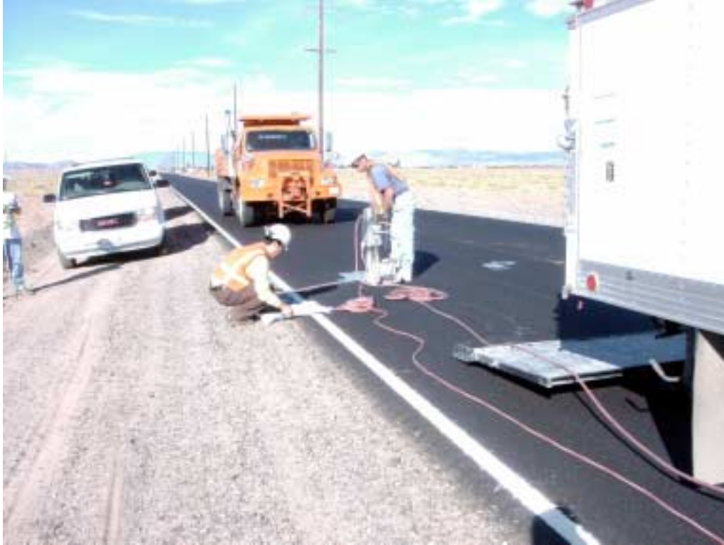
Figure E1. View of coring operation in October, 2002.
