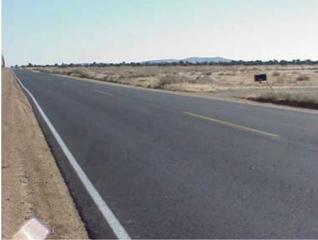
Figure B7. Area of good appearance of levelling course DGAC.
