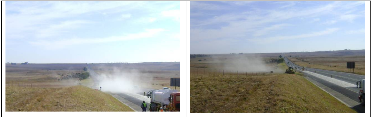
Figure 7.2: Cement loss by wind.
