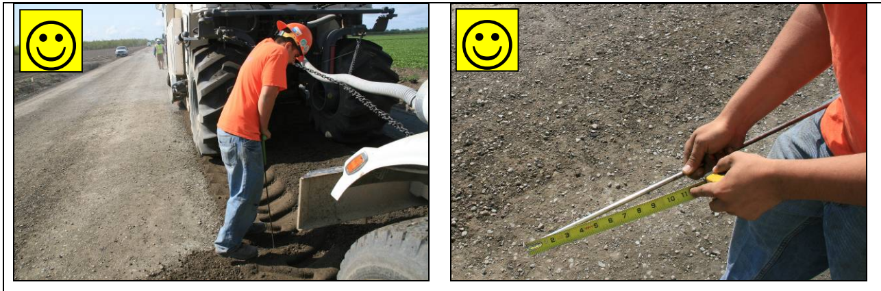
Figure 7.5: Checking mixing depth.
