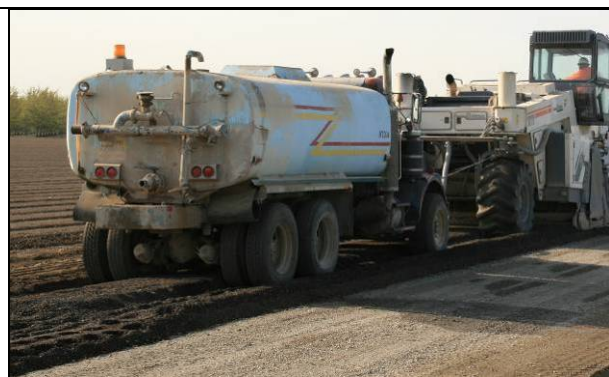
(a) Rotary mixer/recycler coupled to water tanker
