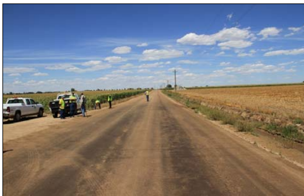
Figure 2.6: Road treated with lignosulfonate.
