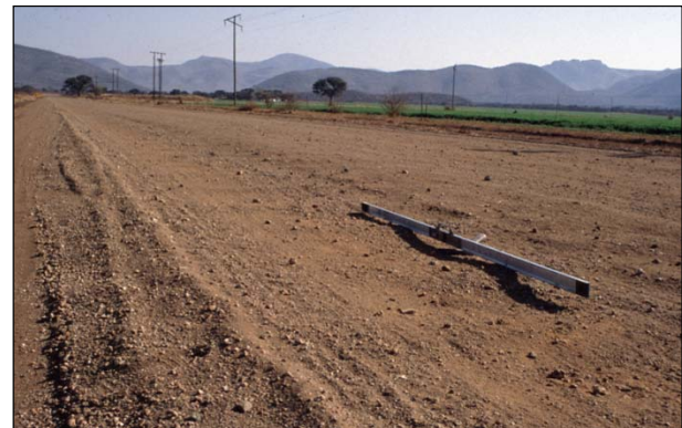
Figure B.12: Washboarding and raveling.
