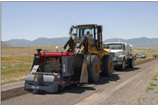
Figure 5.16: Equipment-mounted recycler.
