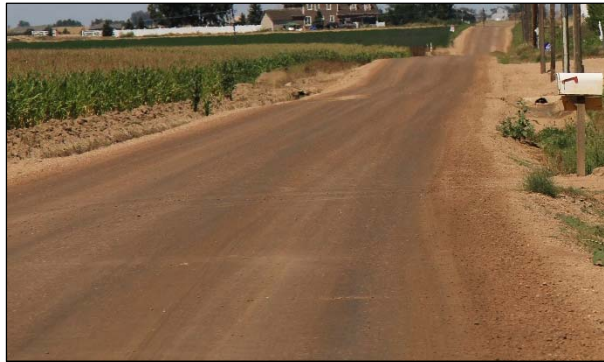
Figure 2.8: Road treated with petroleum resin.
