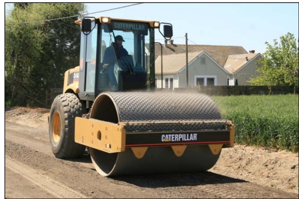
Figure 5.21: Compaction with a smooth-drum roller.
