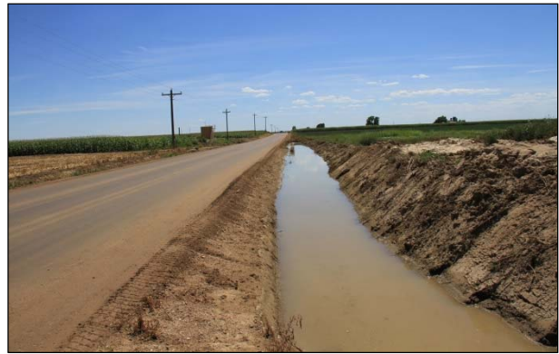
Figure 5.10: Water ponding next to road.
