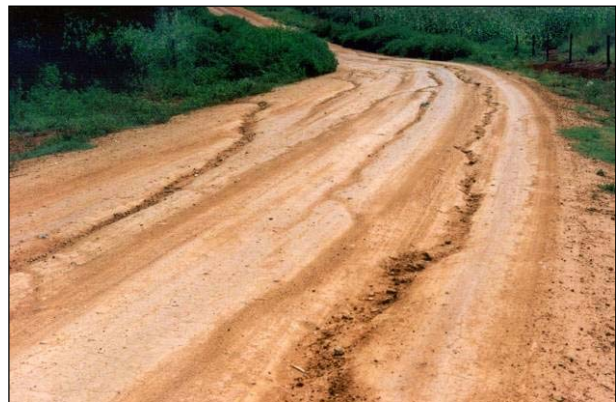
Figure B.9: Longitudinal erosion.
