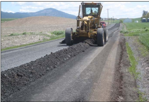
Figure 5.20: Shaping the road.
