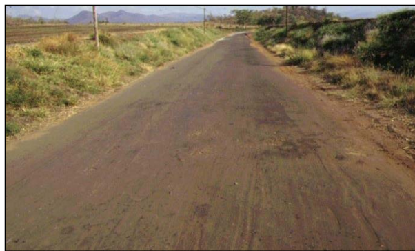
Figure 2.7: Road treated with asphalt emulsion.
