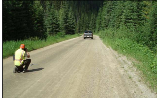
Figure 2.4: Road treated with magnesium chloride.
