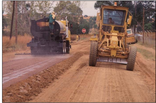
Figure 5.25: Blade mixing application.
