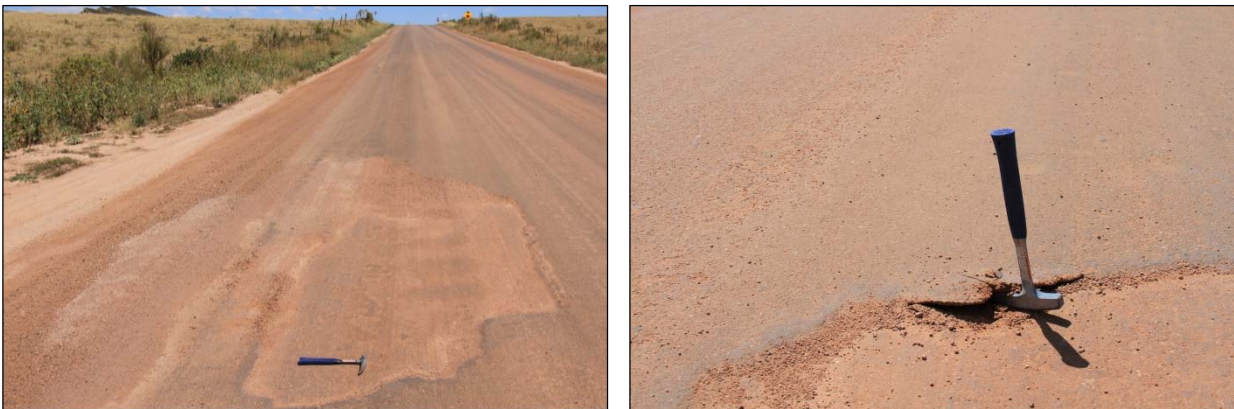
Figure 5.4: Effect of biscuit layer on treated surface.
