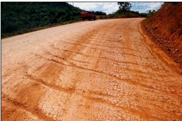
Figure B.8: Transverse erosion.
