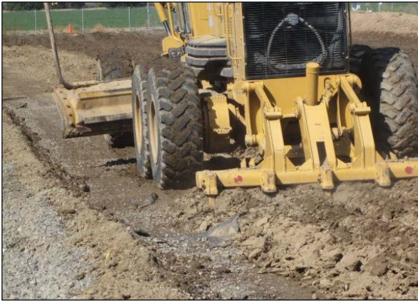
Figure 5.18: Ripping with a grader.
