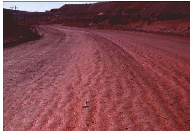
Figure 2.2: Erosion caused by repeated water spraying.
