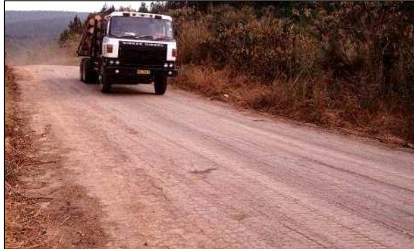
Figure 2.11: Road treated with concentrated liquid stabilizer.
