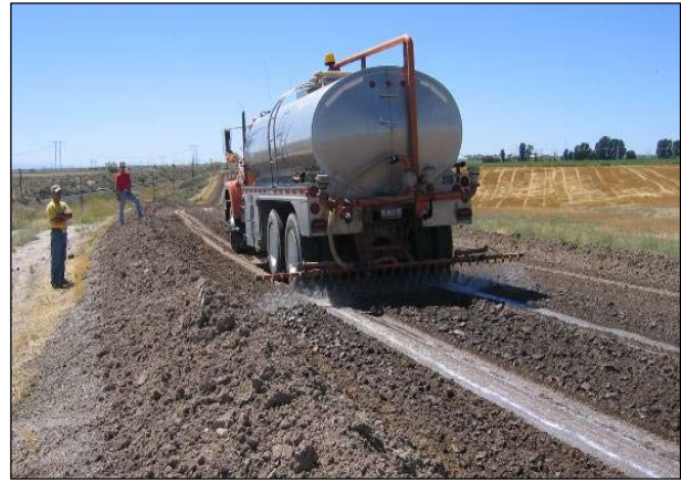
Figure 5.19: Spraying the chemical treatment.
