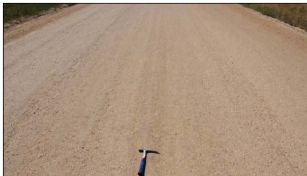
Figure 2.10: Road treated with synthetic polymer emulsion.
