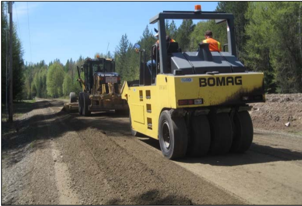
Figure 5.22: Compaction with a rubber-tired roller.
