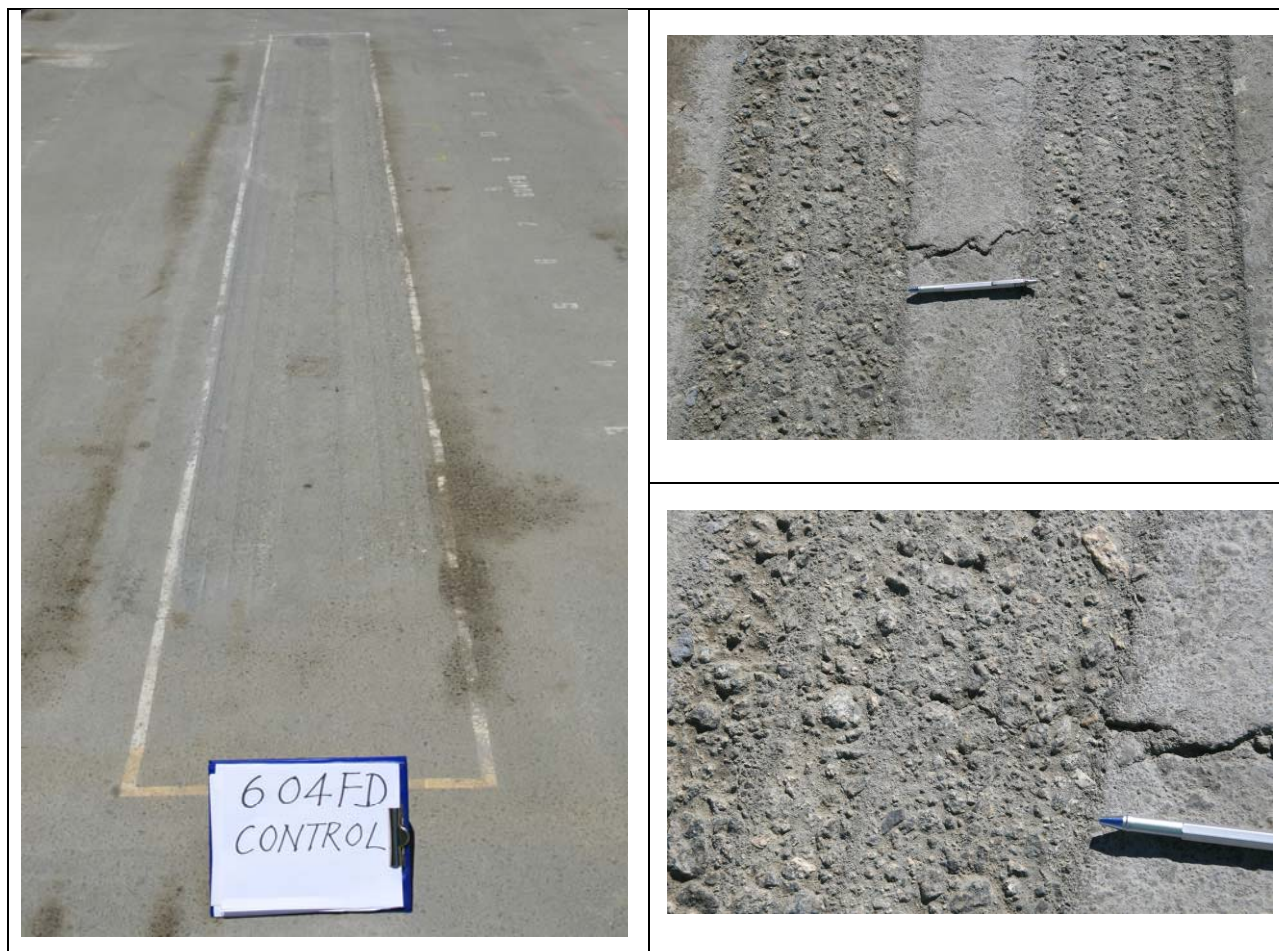
Figure 4.18: 604FD: Section photographs at test completion.
