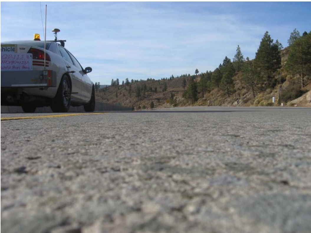
Figure A.8: Longitudinally broomed, OBSI=104.1 dB(A) (Section QP-112.3).
