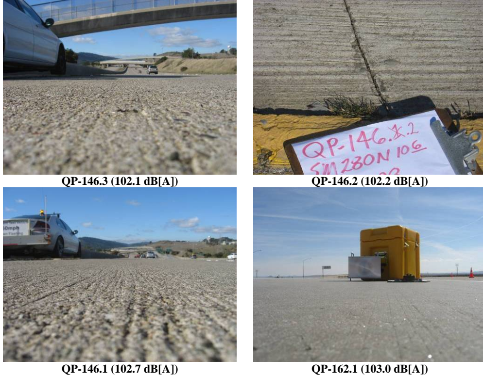
Figure 4.4: Example photographs of longitudinally broomed surfaces and their OBSI levels.
