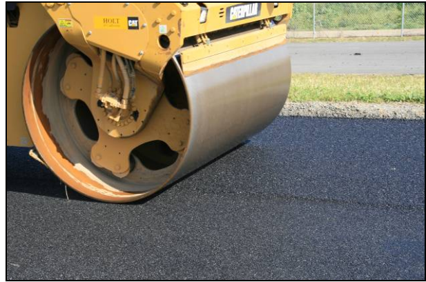
Figure 2.42: Astec: Breakdown rolling.
