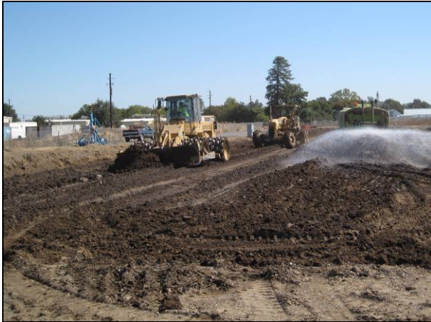
Figure 2.8: Watering and mixing.
