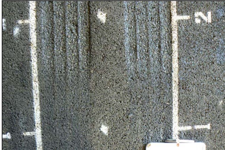
Figure 4.47: 628HB: Section photograph at test completion.
