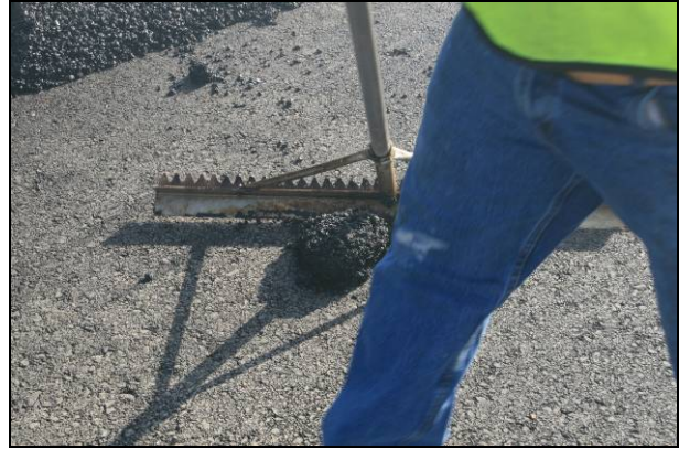
Figure 2.39: Control #2: Chunks removed from section.
