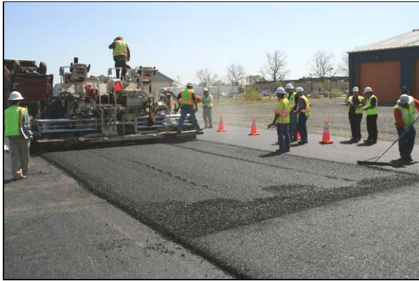
Figure 2.35: Advera: No smoke from truck or paver.
