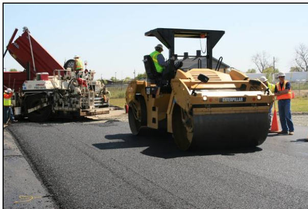
Figure 2.37: Advera: Breakdown rolling.
