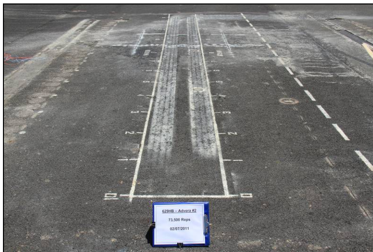
Figure 4.55: 629HB: Section photograph at test completion.
