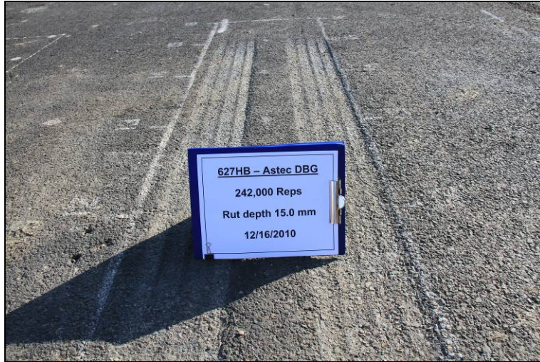
Figure 4.38: 627HB: Section photograph at test completion.
