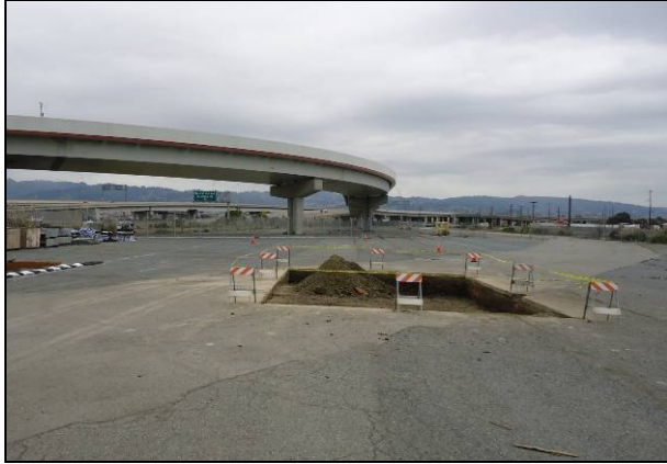
Figure 2.4: Initial excavation.
