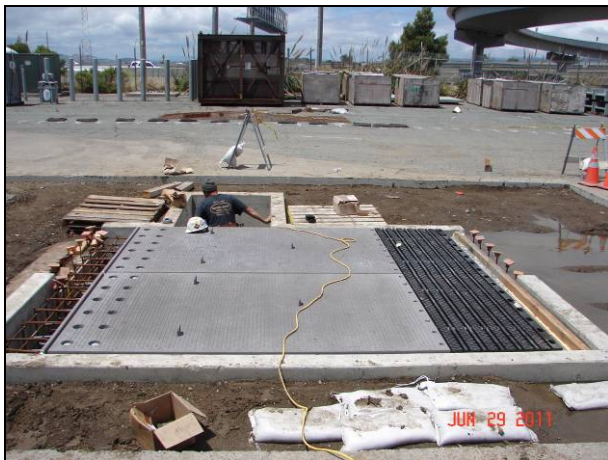
Figure 2.8: Completed steel plate installation.
