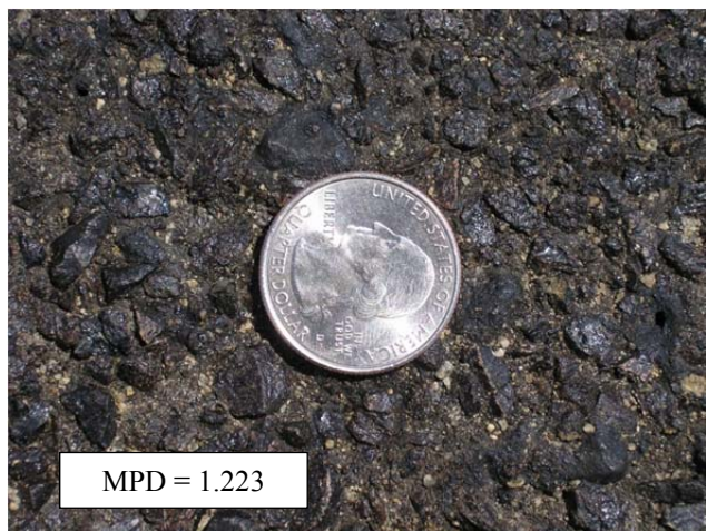
#6 1/4" PME seal coat - double chip seal (PM 10.0-9.8)
