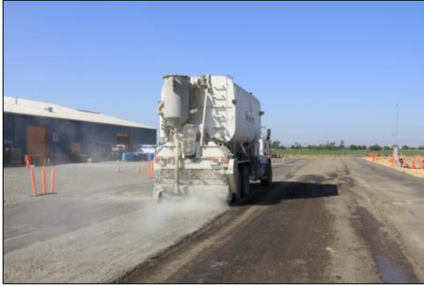
Figure 3.21: FDR-FA: Spreading cement on old asphalt surface.
