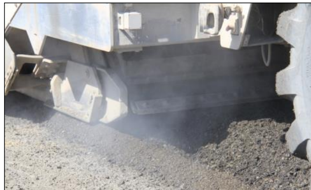
Figure 3.5: FDR-NS: Test track recycling.
