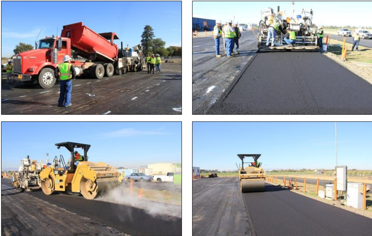
Figure 3.37: Asphalt concrete placement.
