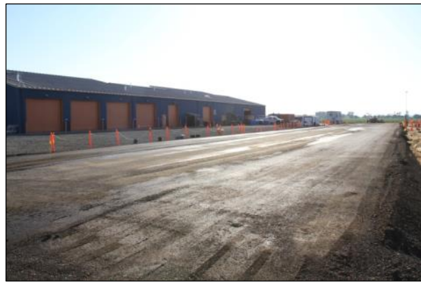
Figure 3.11: FDR-NS: Surface leveling with a grader.
