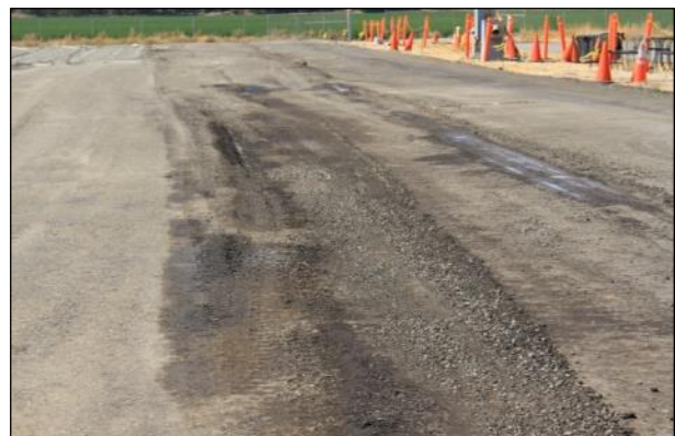
Figure 3.18: FDR-EE: Excess fluid during and after compaction with smooth drum roller.
