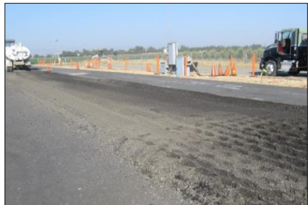
Figure 3.17: FDR-EE: Compaction with padfoot roller. (Note untreated areas and emulsion adhering to tire).
