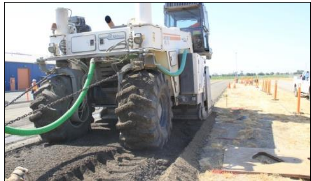
Figure 3.5: FDR-NS: Test track recycling.
