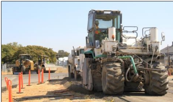
Figure 3.5: FDR-NS: Test track recycling.
