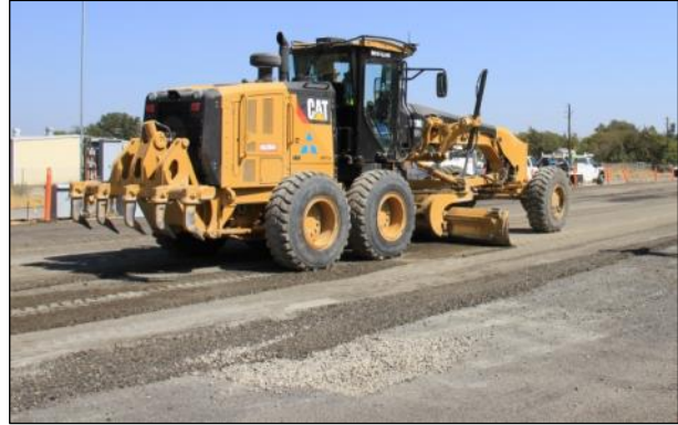
Figure 3.11: FDR-NS: Surface leveling with a grader.
