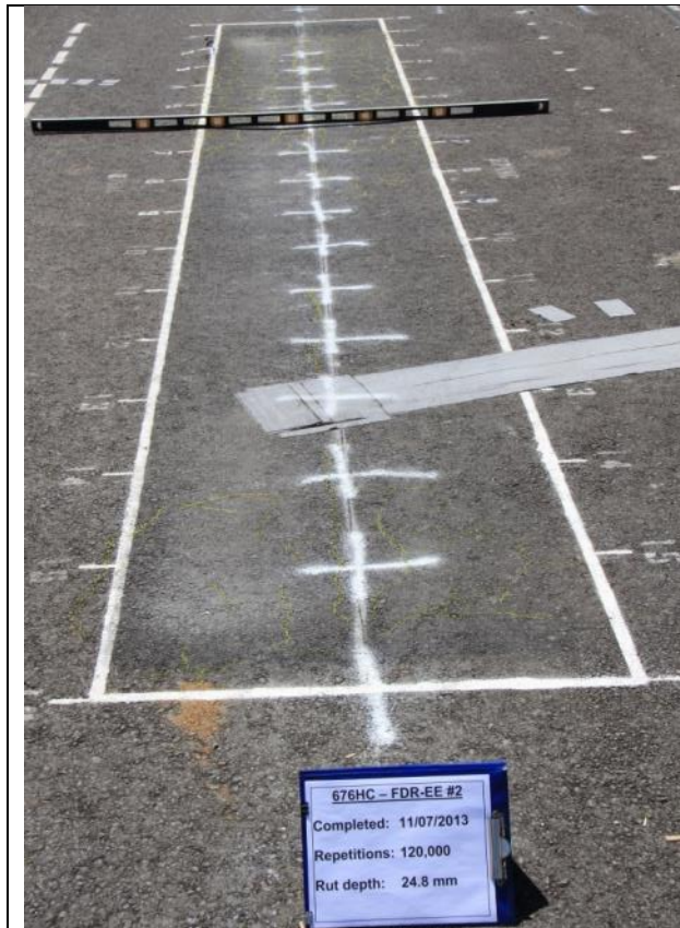
General view of test section looking from east to west
