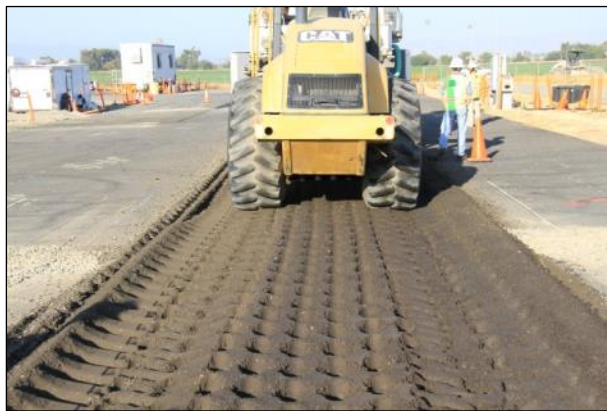
Figure 3.17: FDR-EE: Compaction with padfoot roller. (Note untreated areas and emulsion adhering to tire).
