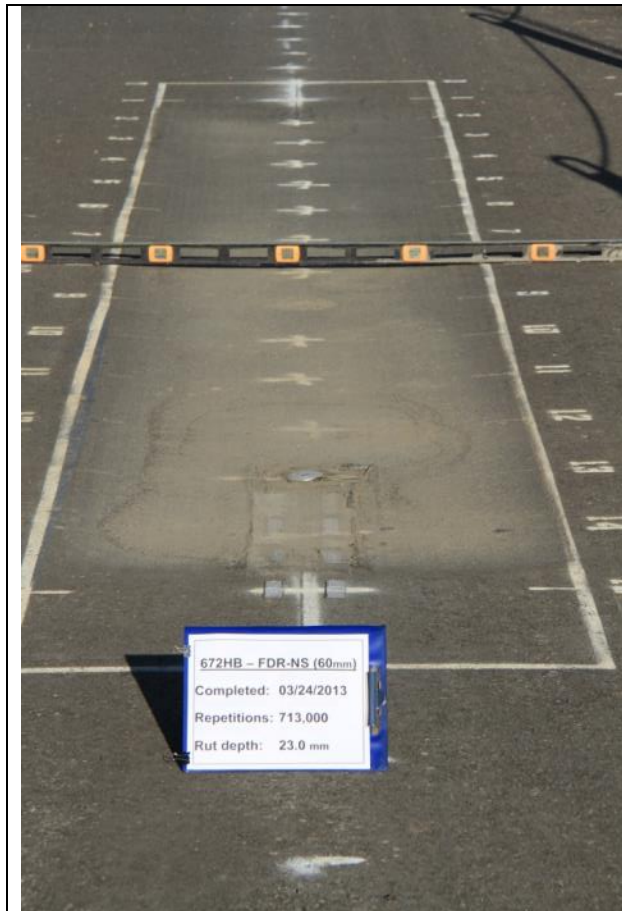
General view of test section looking from east to west
