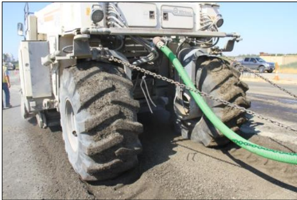
Figure 3.21: FDR-FA: Spreading cement on old asphalt surface.
