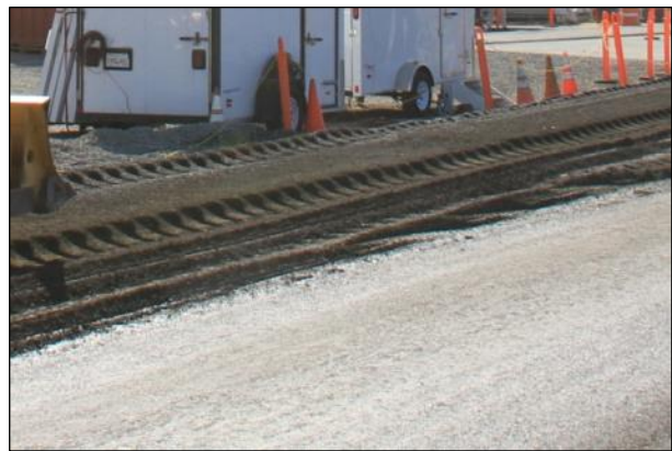
Figure 3.30: FDR-PC: Water spray prior to second mixing pass.
