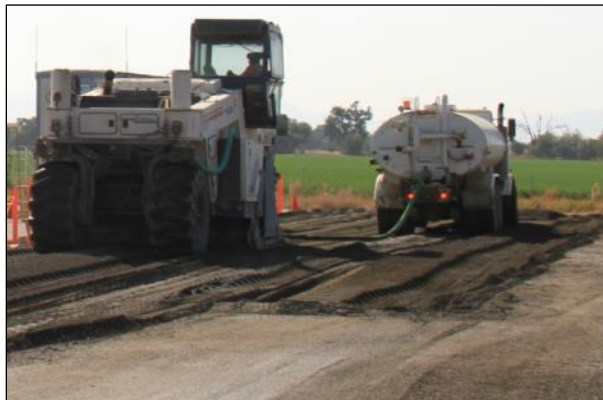
Figure 3.32: FDR-PC: Uniform mix after second recycling pass.
