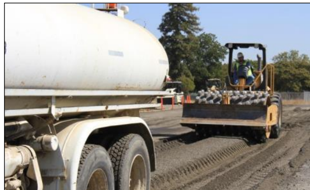
Figure 3.9: FDR-NS: Initial compaction with padfoot roller.
