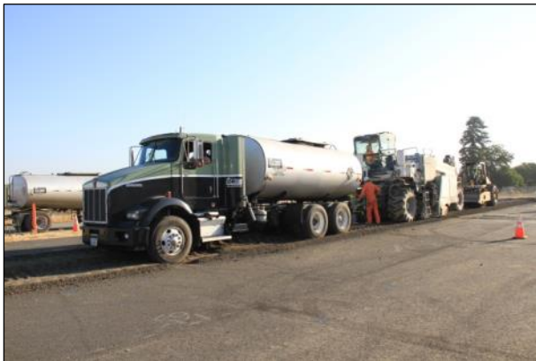
Figure 3.14: FDR-EE: Recycling train.
