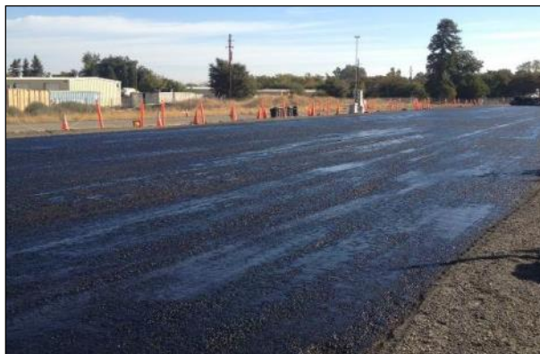
Figure 3.36: Prime coat application.
