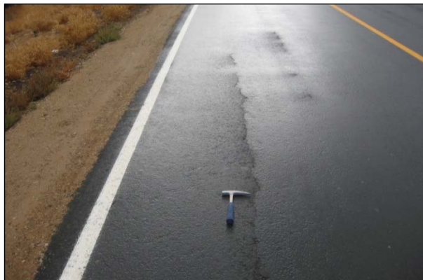
Figure 2.2: Longitudinal crack.
