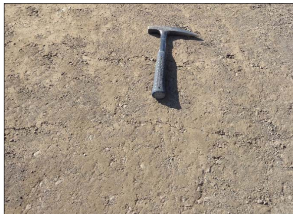
Figure 3.15: CR99: Block cracking after microcracking.
