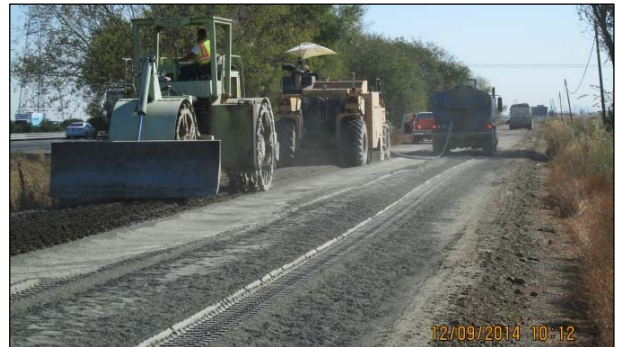
Figure 3.4: CR32B: Water hose dragging on the spread cement.
