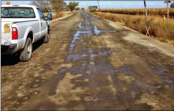
Figure 3.5: CR32B: Surface raveling.
