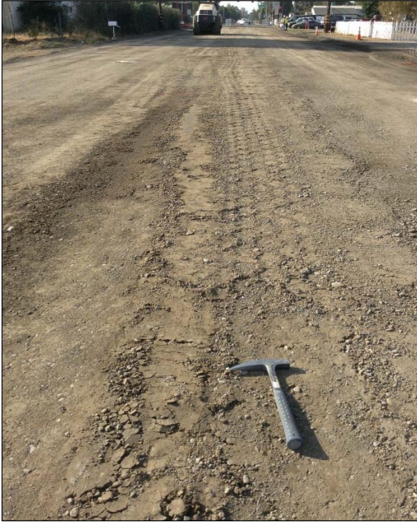
Figure 3.13: CR99: Delamination after microcracking.
