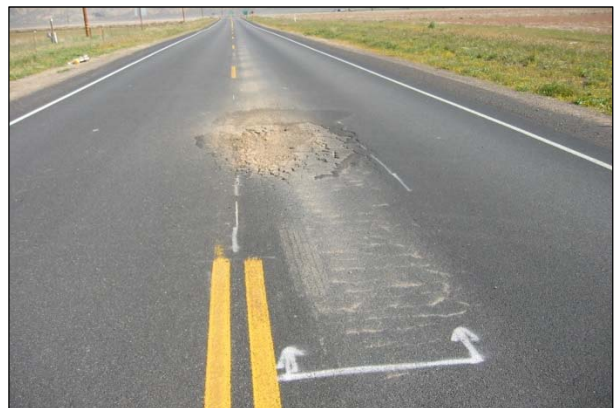
Figure 2.6: Pumping through fatigue cracking.
