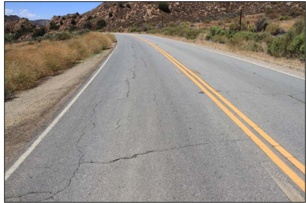
Figure 2.4: Block crack progression.
