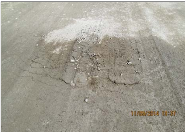
Figure 3.6: CR32B: Wet, soft location after final compaction.
