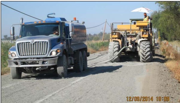
Figure 3.4: CR32B: Water hose dragging on the spread cement.
