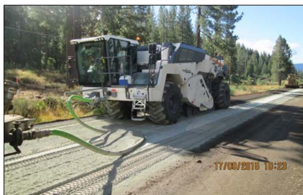
Figure 3.18: PLU147: Water pipe dragging on cement.
