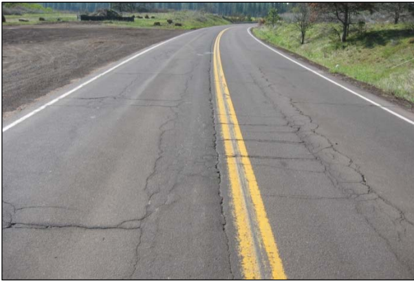
Figure 2.3: Block cracking.
