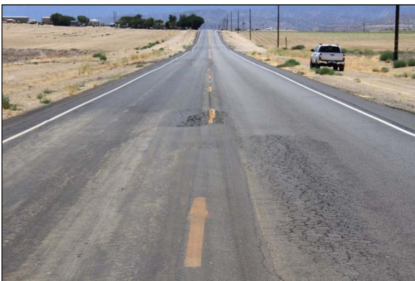
Figure 2.5: Fatigue cracking.
