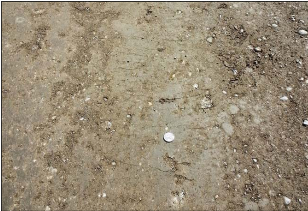
Figure 3.2: CR32B: Transverse cracking after microcracking.
