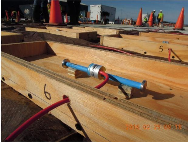
**VWSG inside the mold before placing concrete**
