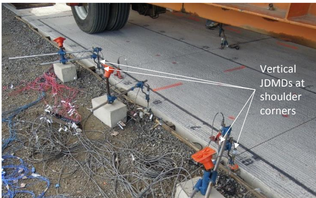
HVS Testing. The structural response under the HVS wheel was measured with dynamic strain gages and JDMDs. In addition to measuring corner deflection, the JDMD readings were used to determine the load transfer efficiency (LTE) of the transverse joints under the passing HVS wheel.
