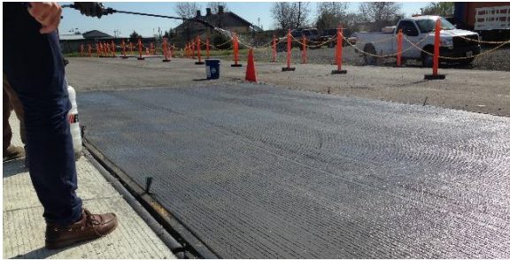
Application of topical SRA Spray. SRA was applied right after the “shine” on the concrete surface disappeared. The timing matches that for the application of standard curing compound.
