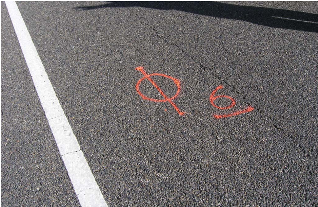
Figure 6: Lake 53 longitudinal crack in the wheelpath (PM 4.0 SB, near Olympic Dr.).
