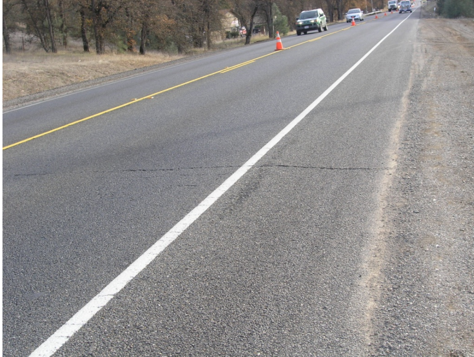
Figure 7: Lake 53 transverse crack (near PM 5.25 NB).
