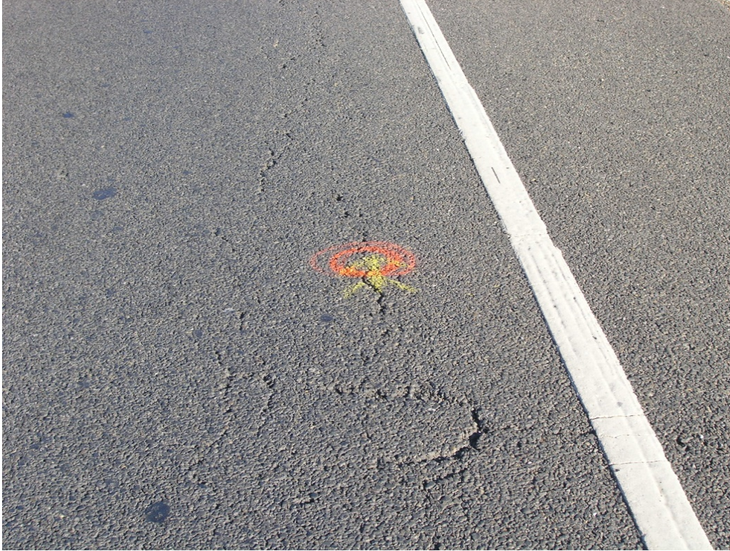
Figure 5: Lake 53 Alligator B crack in the wheelpath (PM 3.3 NB, north of Davis Ave.).
