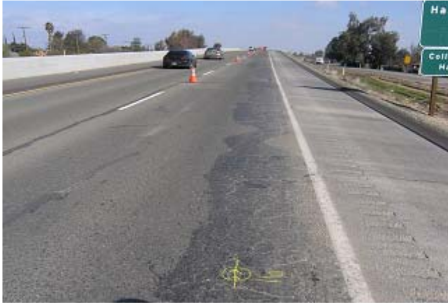
Figure 4: Photo shows sealant over Alligator B cracking on an embankment, Section 2 near PM 14.7 EB.
