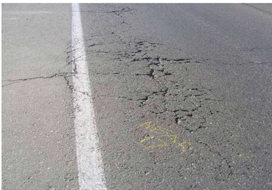
Figure 3: Alligator cracking in the wheelpath with transverse cracking, Section 3 near PM 15.2 EB.
