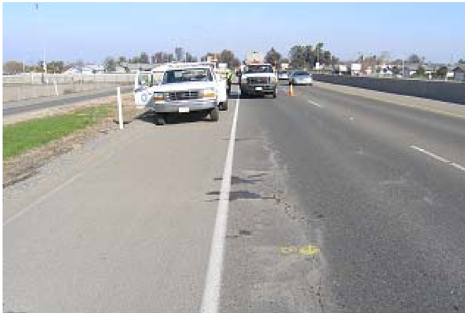
Figure 5: Fines pumped through longitudinal cracking are visible, Section 3 near PM 15.1 WB.
