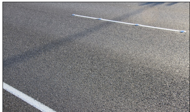
Figure 5.4: Orland Evotherm, June 2011 (24 months). Note ruts in wheelpath.
