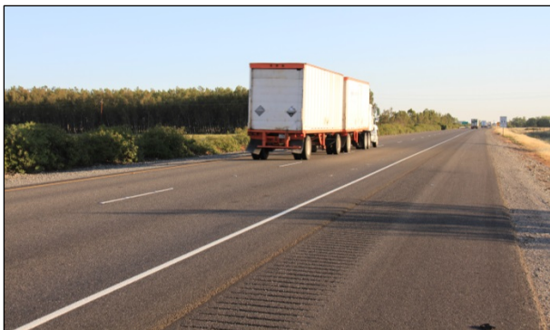
Figure 5.4: Orland Evotherm, June 2011 (24 months). Note ruts in wheelpath.
