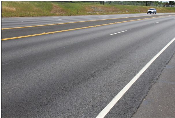
Figure 8.3: Auburn Evotherm, July 2012 (24 months). Note deterioration and reflected crack.
