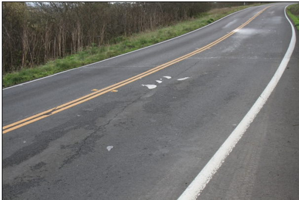
Figure 4.3: Point Arena Evotherm, November 2010, showing longitudinal cracks.
