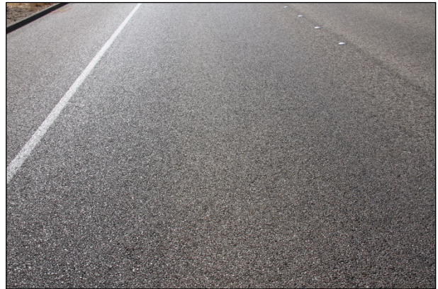
Figure 3.3: Morro Bay Control, May 2012 (60 months), track marks no longer visible.
