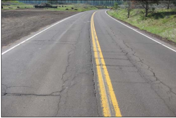
Figure 2.3: Block cracking.
