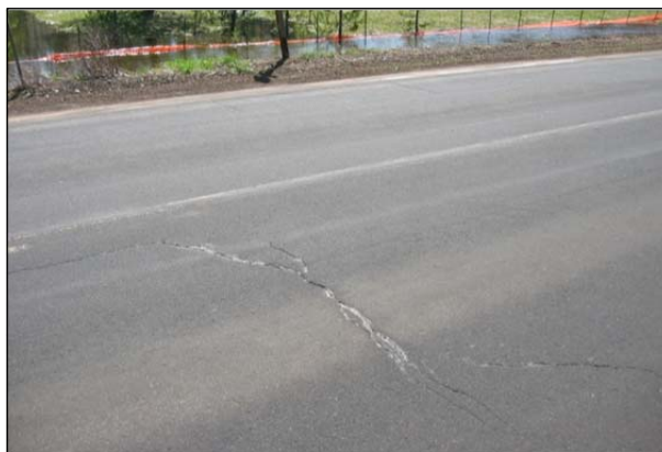
Figure 2.1: Transverse crack.
