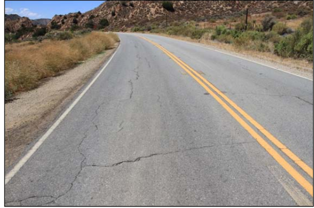
Figure 2.4: Block crack progression.
