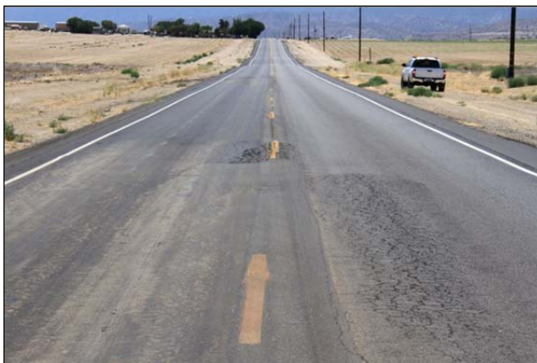
Figure 2.5: Fatigue cracking.
