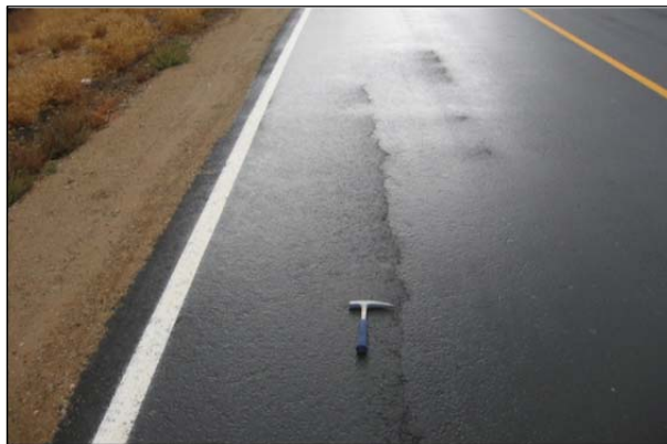
Figure 2.2: Longitudinal crack.
