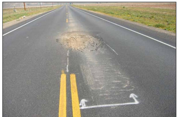
Figure 2.6: Pumping through fatigue cracking.
