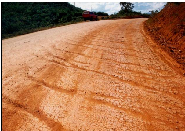
Figure 4: Transverse erosion.
