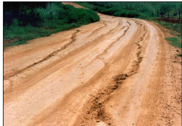
Figure 5: Longitudinal erosion.
