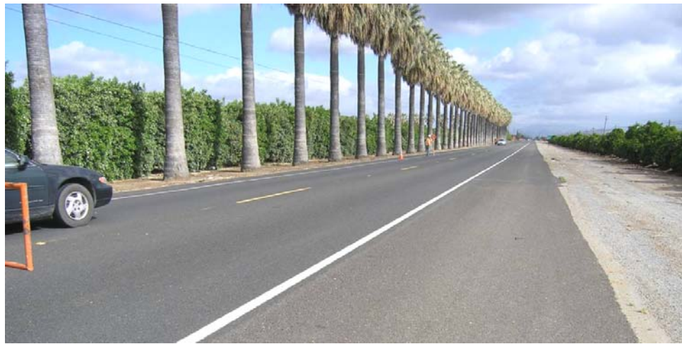
Figure 2.9. One of the 76 roads included in the UCPRC pavement noise study, started in 2006 in California.
