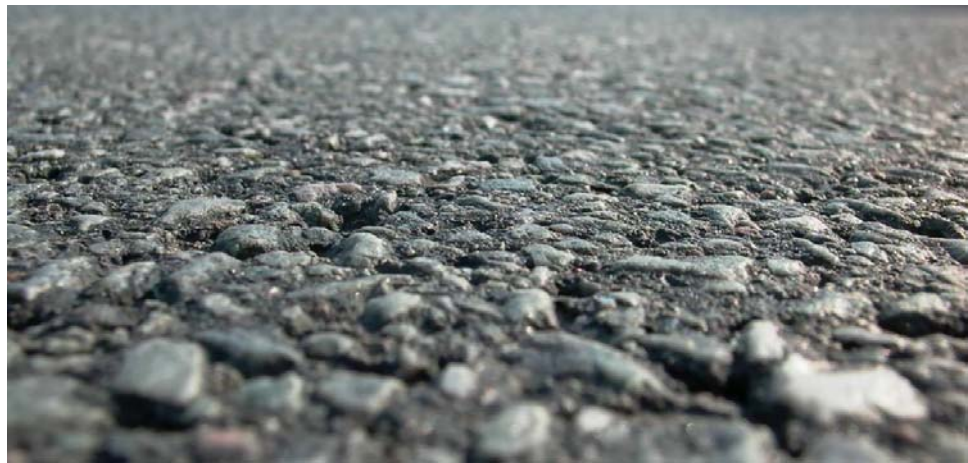
Figure 1.10. A three years old dense-graded asphalt concrete (DGAC) where the bitumen film has been worn off and where no significant signs of wear and tear and distress can be observed.
