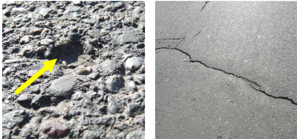
Figure 1.11. Raveling, loss of aggregate (to the left) and cracking (to the right).
