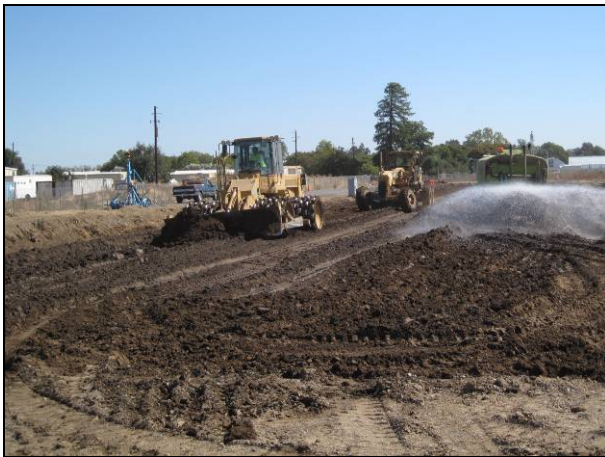
Figure 2.8: Watering and mixing.
