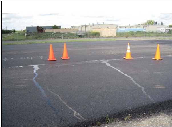
Figure 2.49: Water seepage from longitudinal joint between Cecabase and Control sections.
