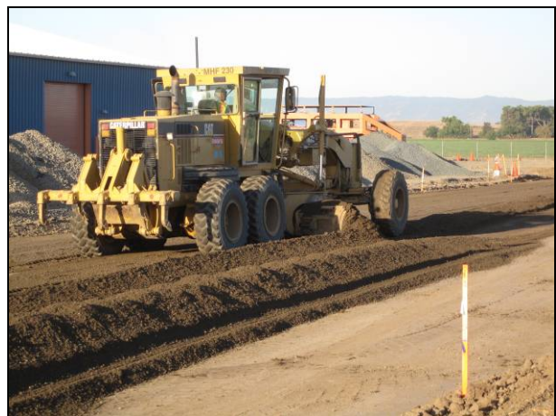
Figure 2.16: Material spreading.
