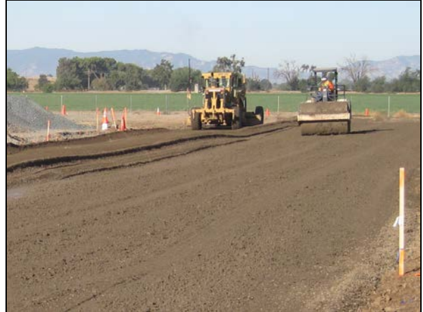
Figure 2.18: Initial compaction.
