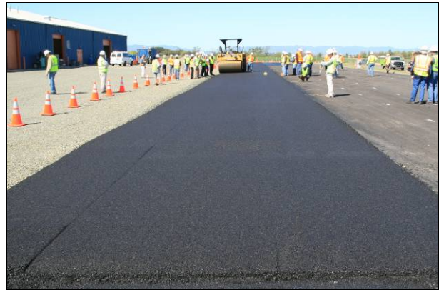
Figure 2.35: Evotherm: Breakdown rolling.
