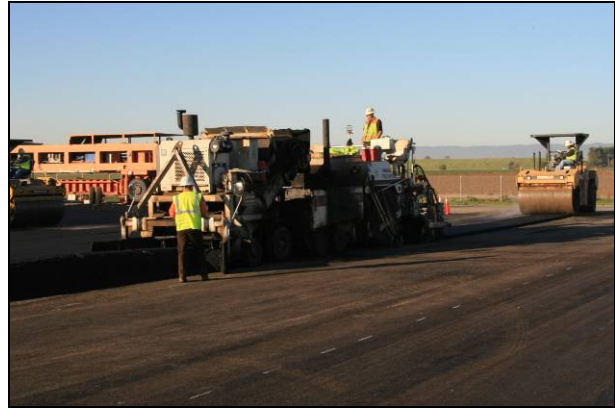
Paving and breakdown rolling
