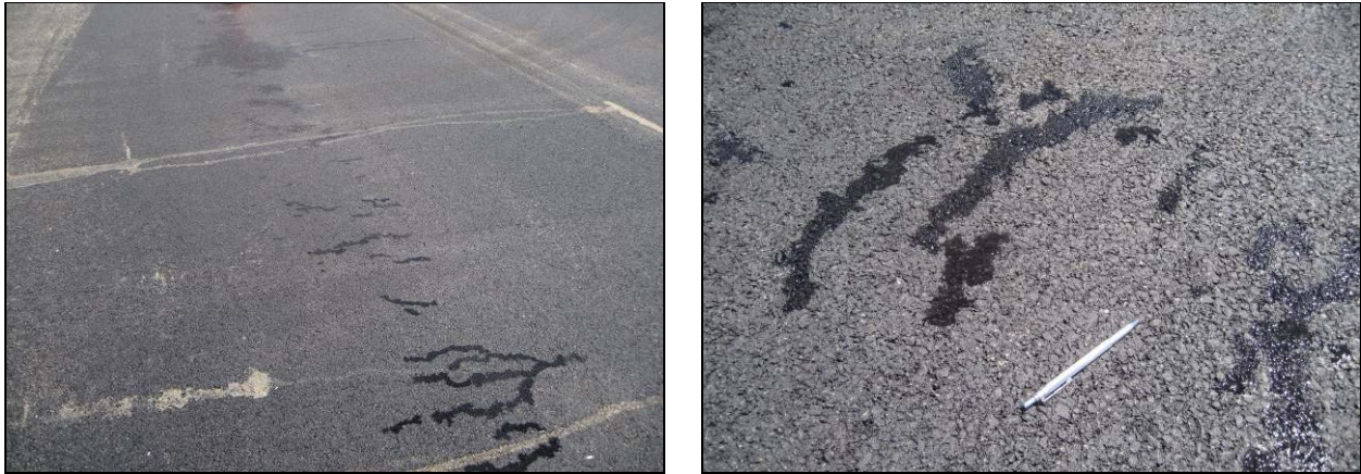
Figure 2.48: Water seepage from Cecabase section.
