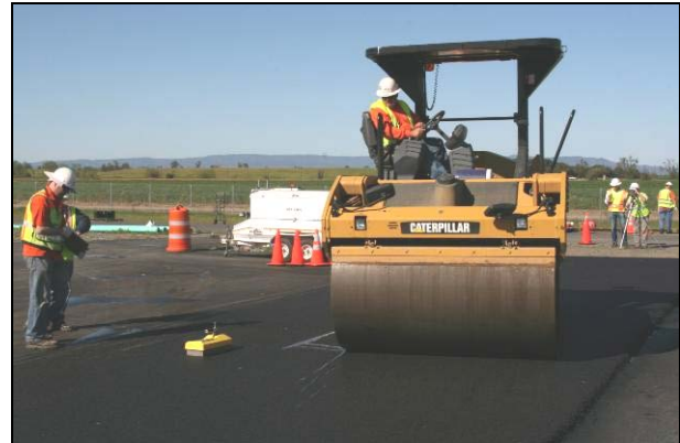
Figure 2.31: Control: Final rolling.
