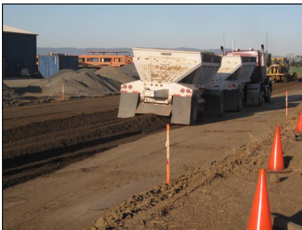
Figure 2.15: Dumping material in windrows.
