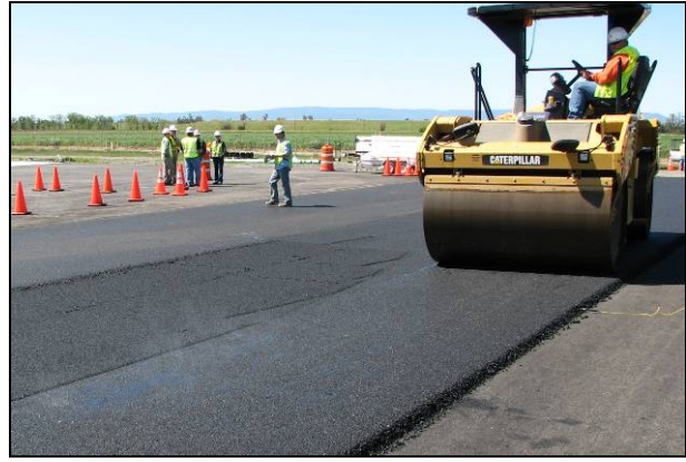
Figure 2.38: Cecabase: Breakdown rolling.
