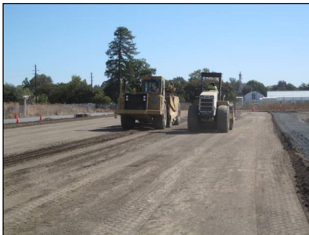
Figure 2.19: Heavy watering prior to pre-final compaction.
