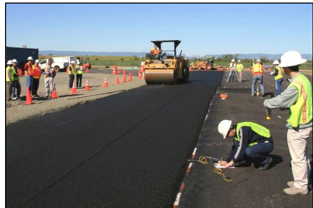
Figure 2.33: Gencor: Breakdown rolling.
