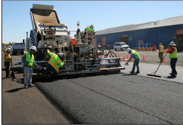
Figure 2.37: Cecabase: No smoke from truck and paver.
