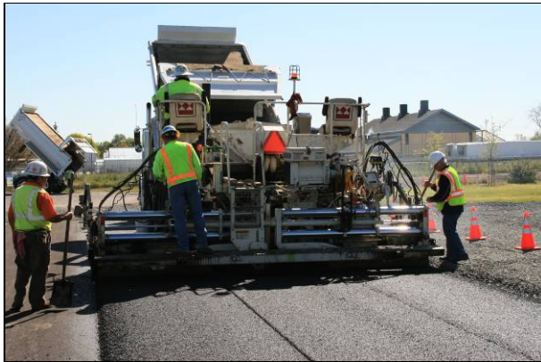
Figure 2.34: Evotherm: No smoke from truck and paver.
