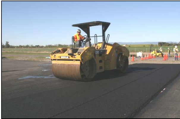
Figure 2.30: Control: Breakdown rolling.
