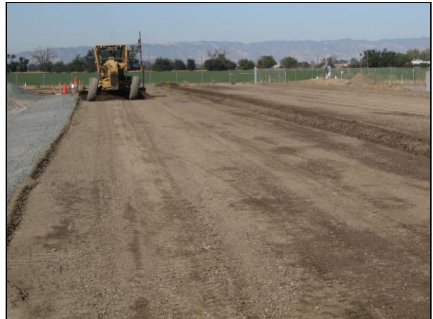
Figure 2.18: Initial compaction.
