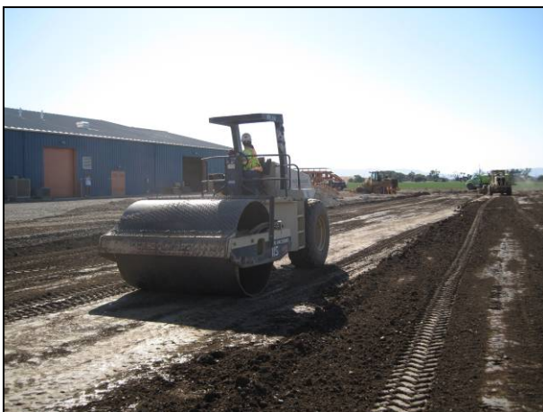
Figure 2.12: Final compaction.
