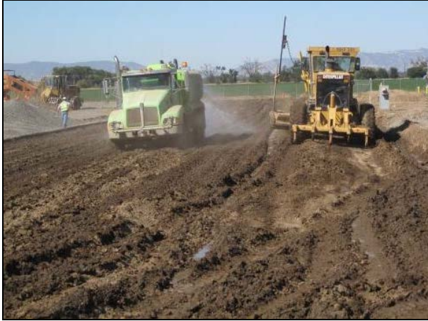
Figure 2.8: Watering and mixing.
