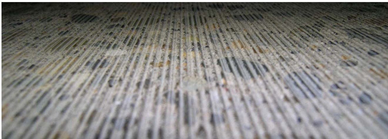
Figure 3.2: Concrete surface after the Next Generation Lite (NGL) grind.
