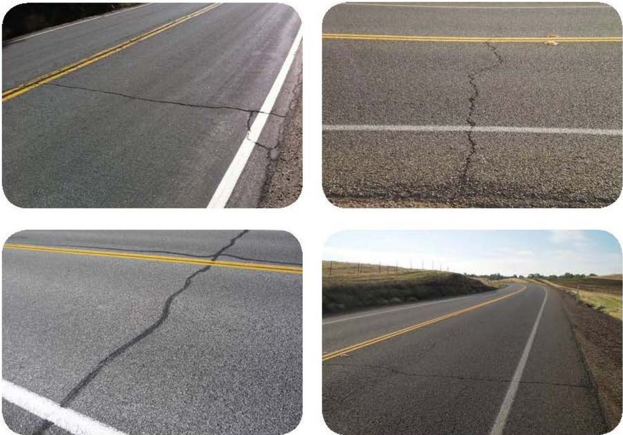
Figure 3-6. Examples of transverse crack.
