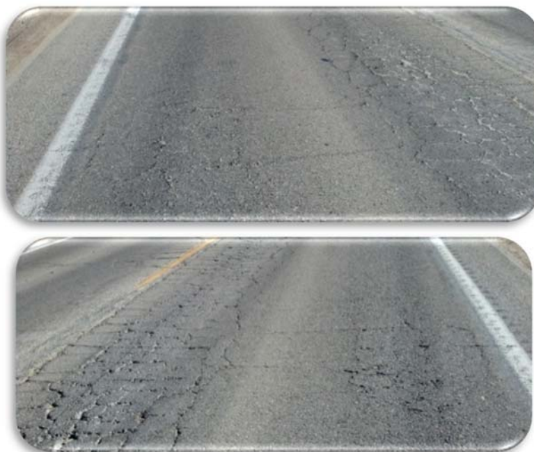
Figure 3-2: Example of alligator B cracking.
