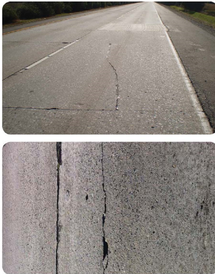
Figure 4-2. Examples of longitudinal cracks.
