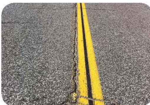
Figure 3-5. Examples of longitudinal cracks.
