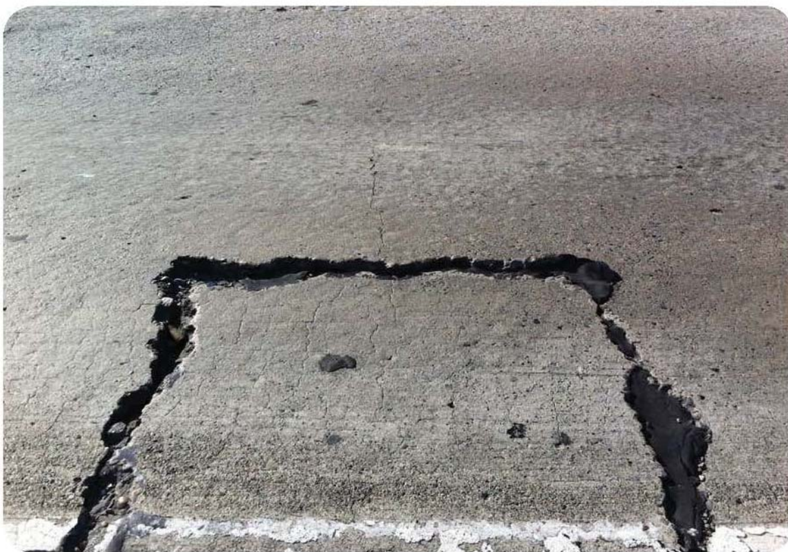
Figure 5-3. Examples of punchout.
