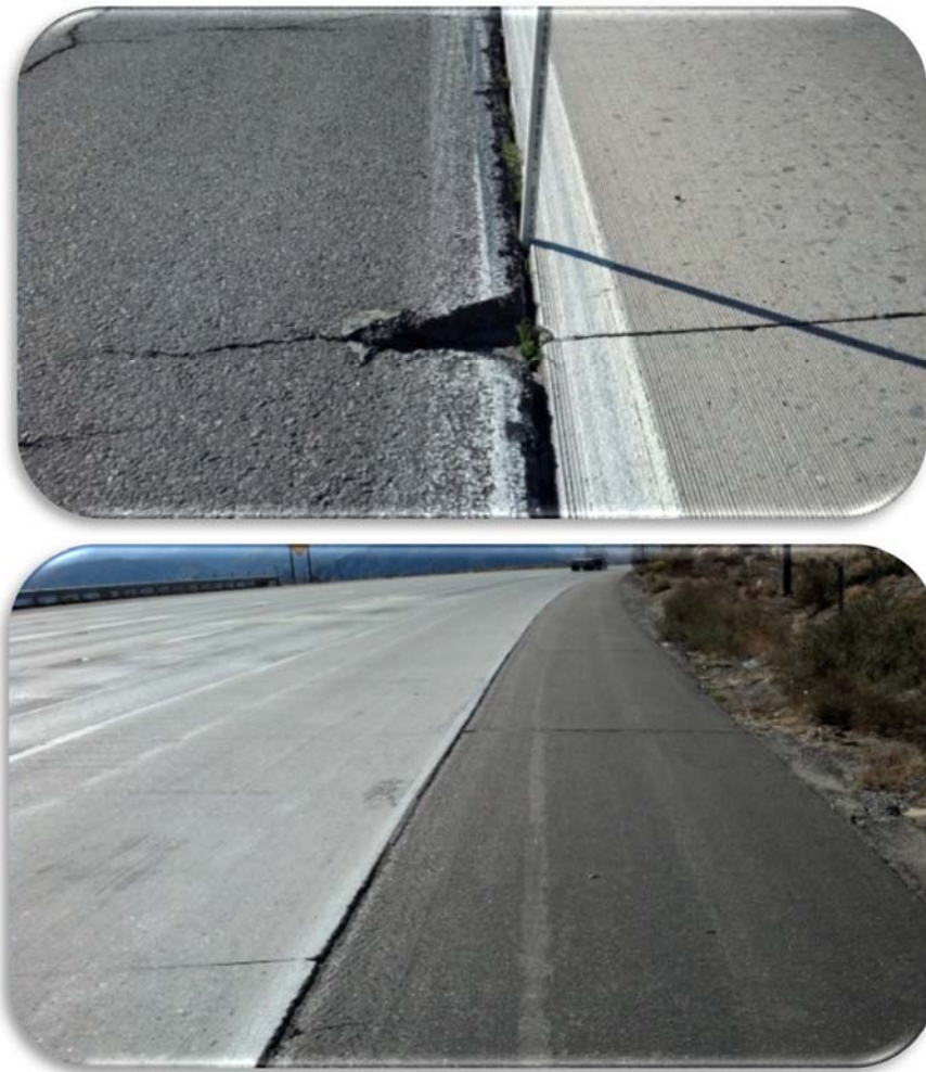
Figure 4-7. Examples of lane/shoulder crack width.
