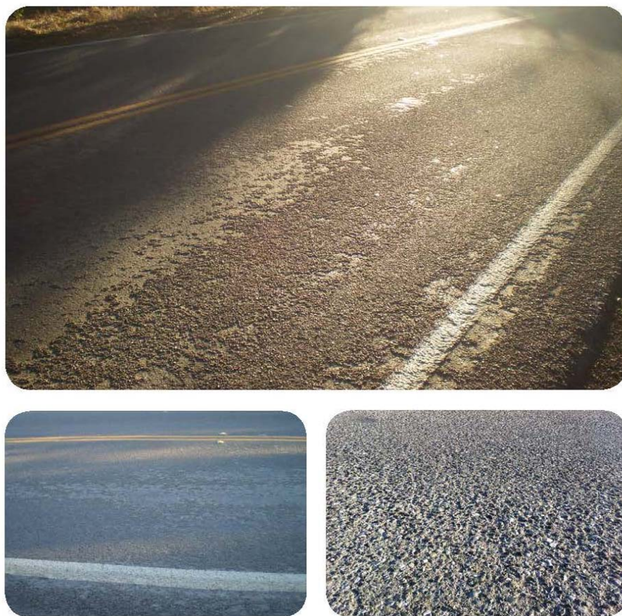
Figure 3-9. Examples of raveling.
