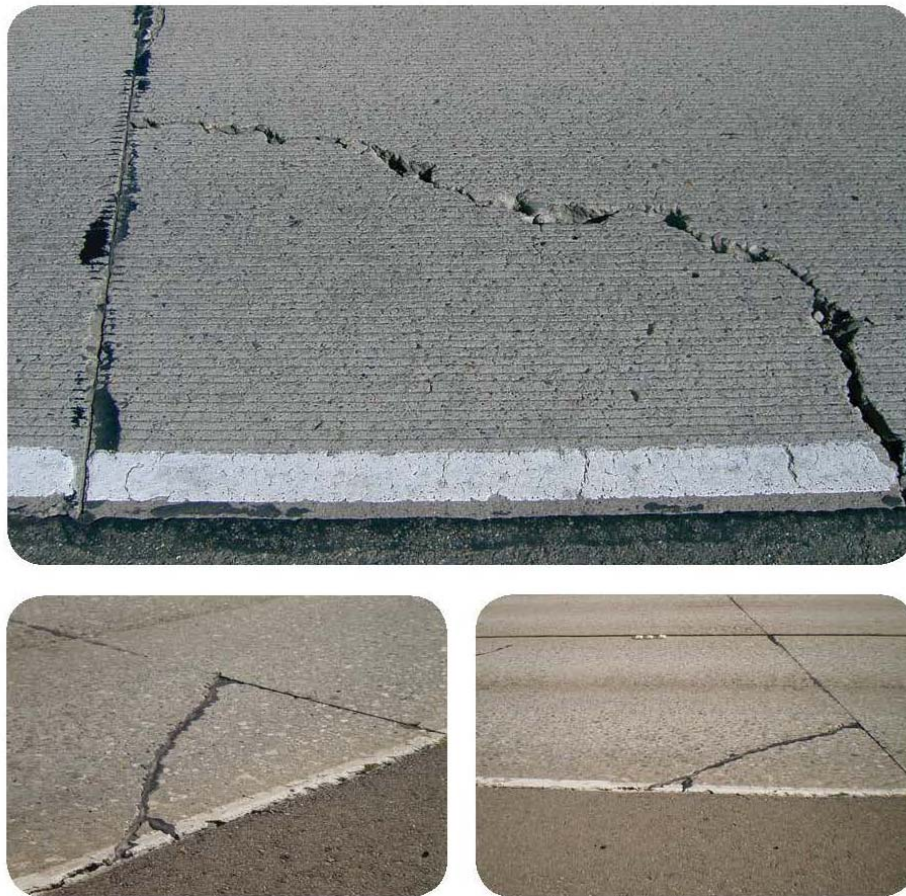
Figure 4-1. Examples of corner cracks
