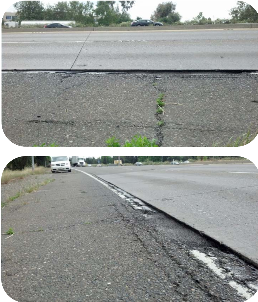
Figure 4-6. Examples of lane/shoulder drop-off.
