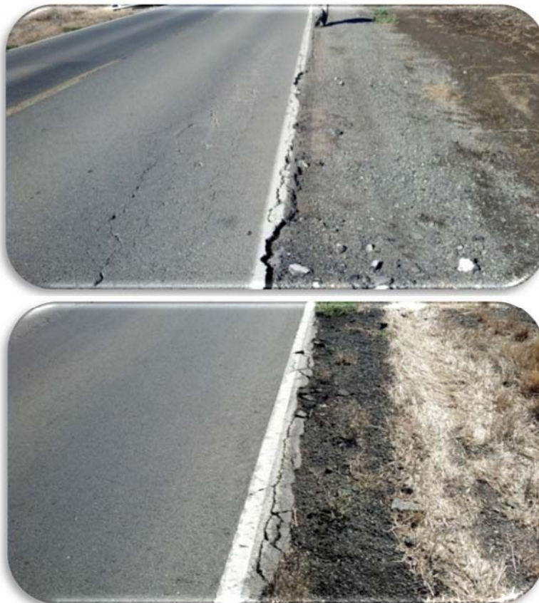
Figure 3-4. Examples of edge cracking.
