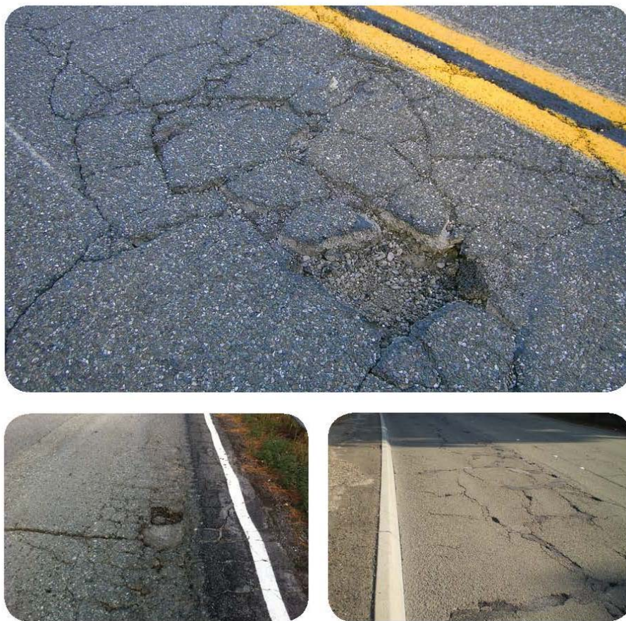
Figure 3-7. Examples of pothole.
