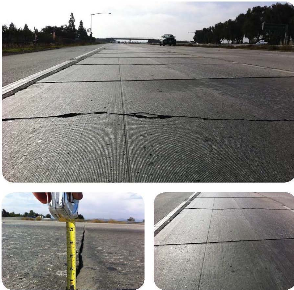
Figure 6-3. Examples of faulting.
