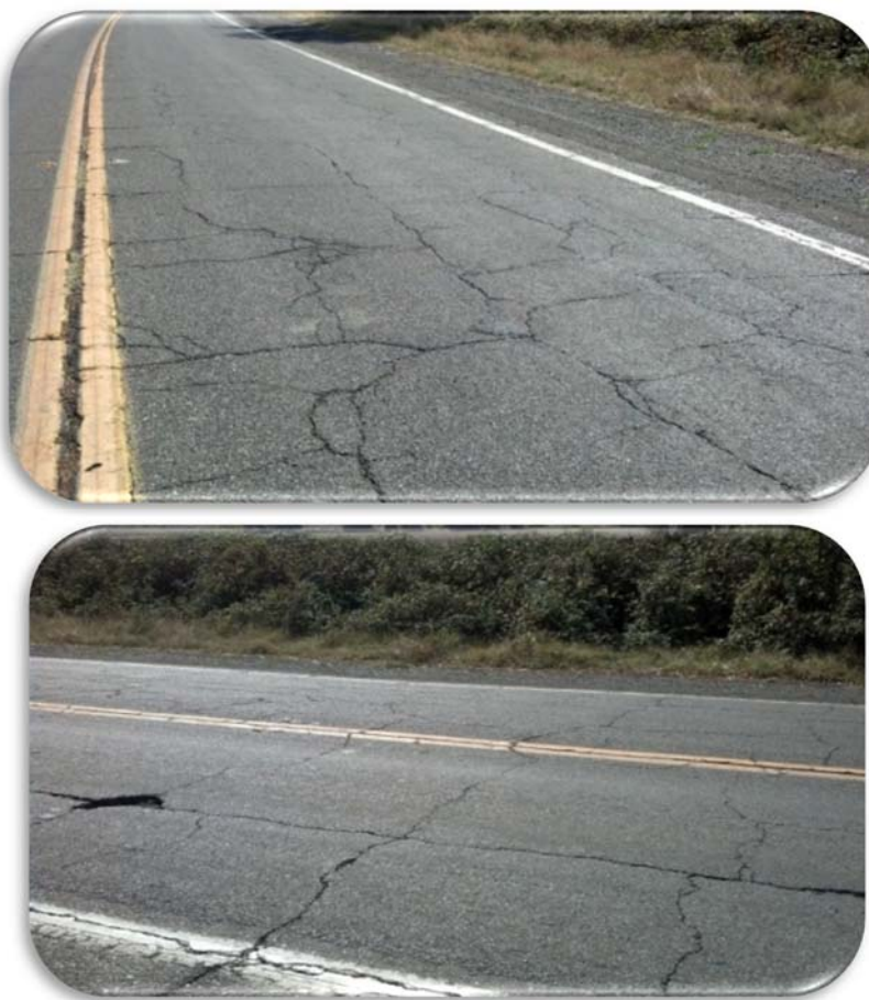
Figure 3-3. Examples of block cracking.
