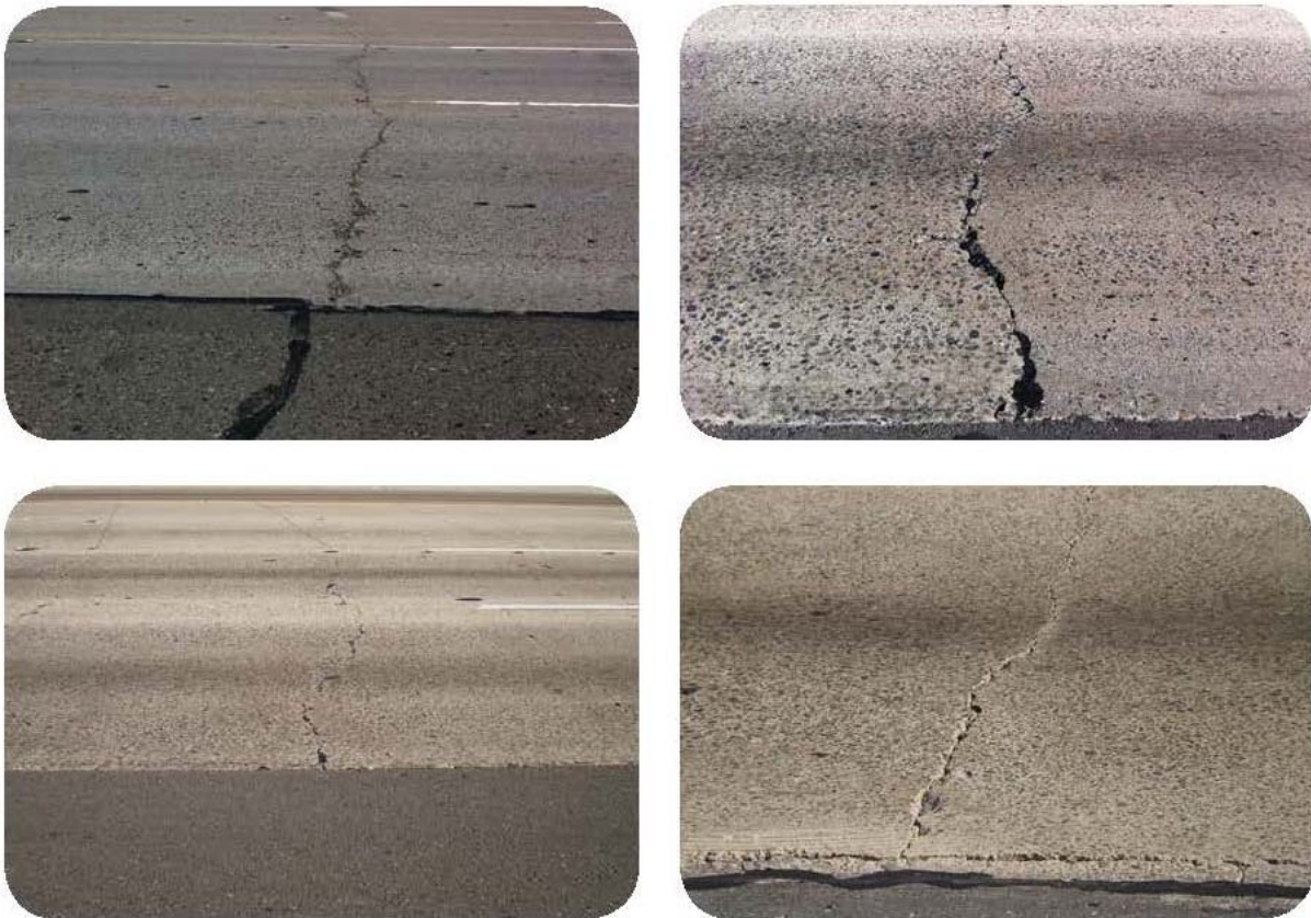
Figure 5-2. Examples of transverse cracks.
