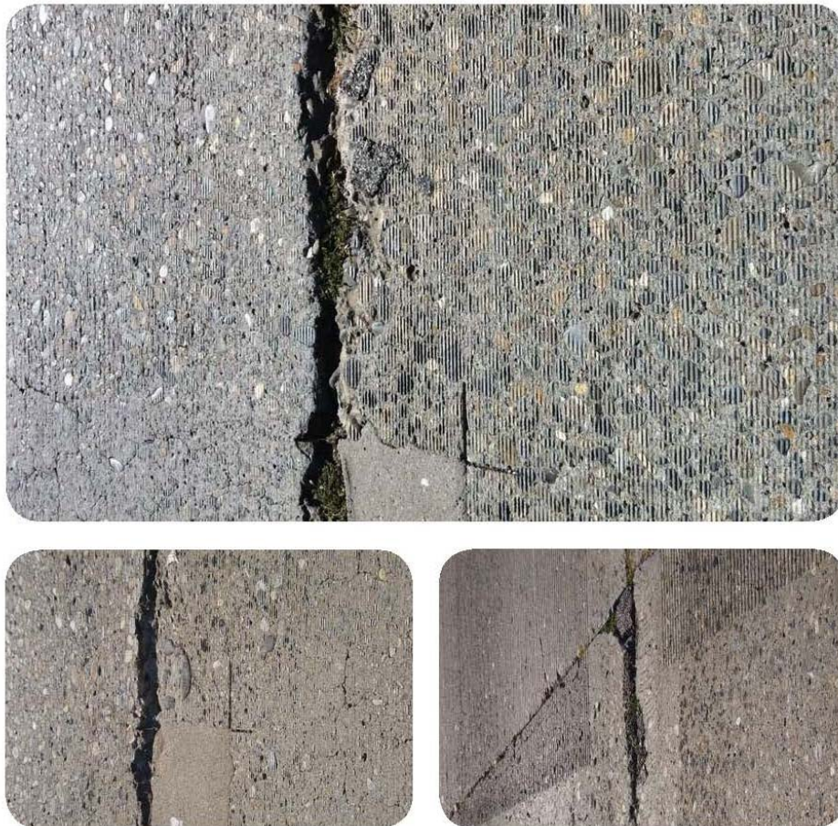
Figure 4-4. Examples of joint spalling.
