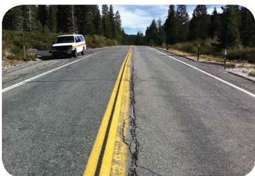
Figure 3-5. Examples of longitudinal cracks.
