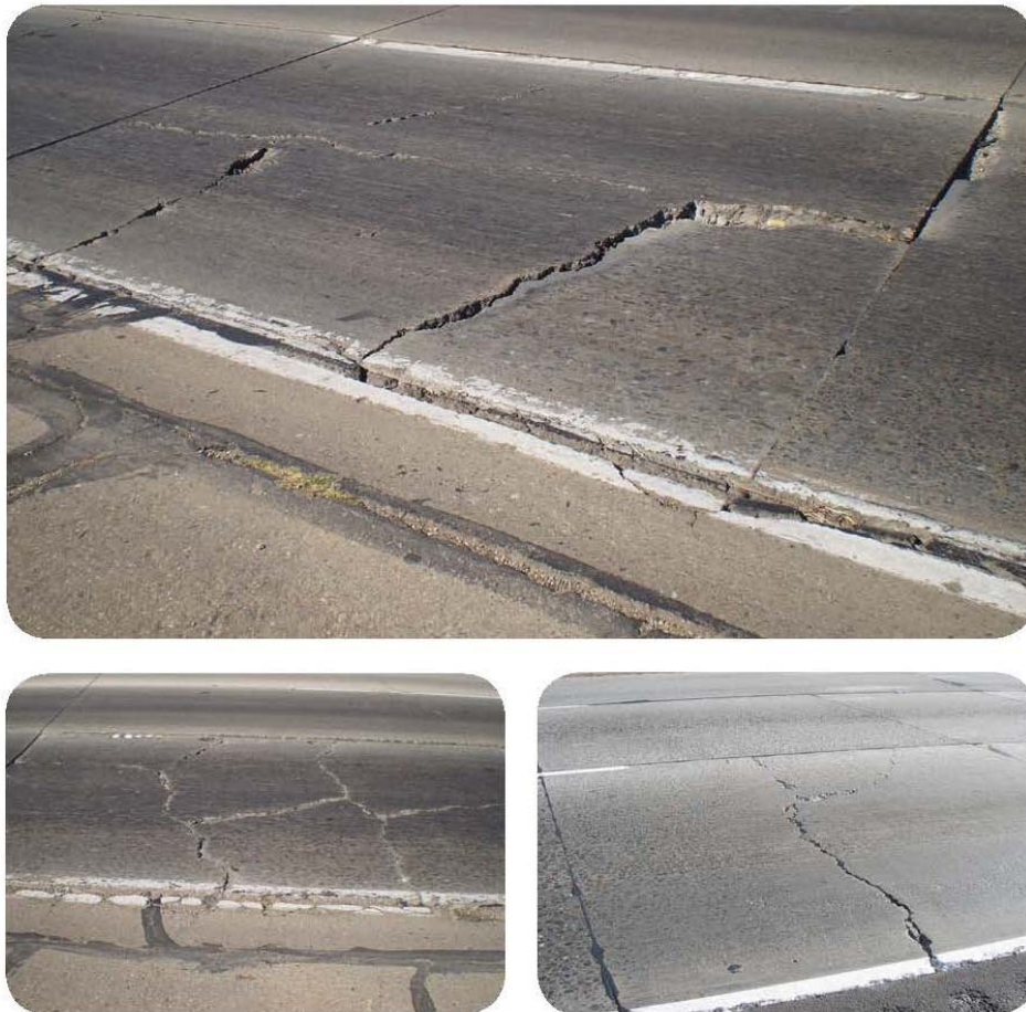
Figure 4-5. Examples of third stage cracking.
