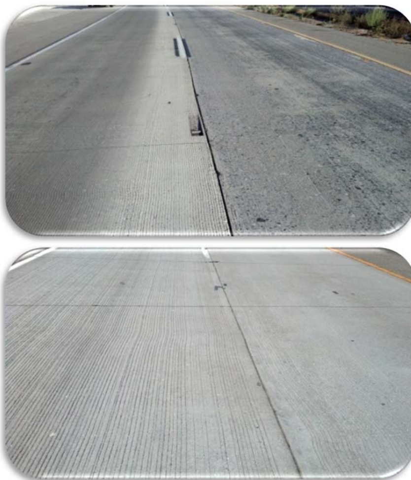
Figure 4-8. Examples of longitudinal joint.
