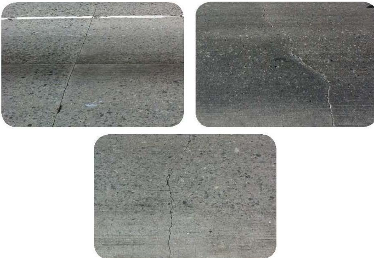
Figure 4-3. Examples of transverse cracks.
