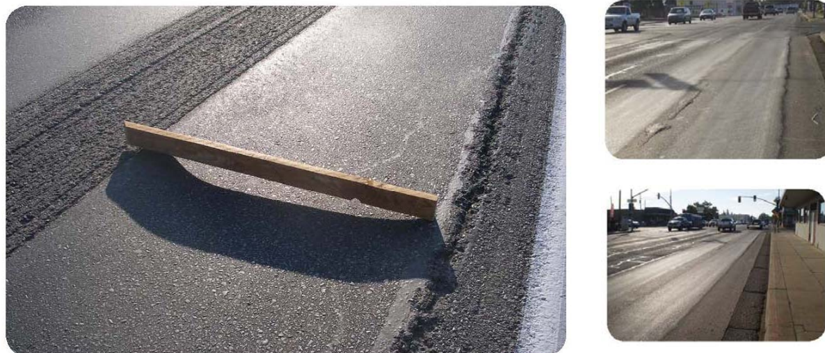
Figure 6-1. Examples of rutting in asphalt.
