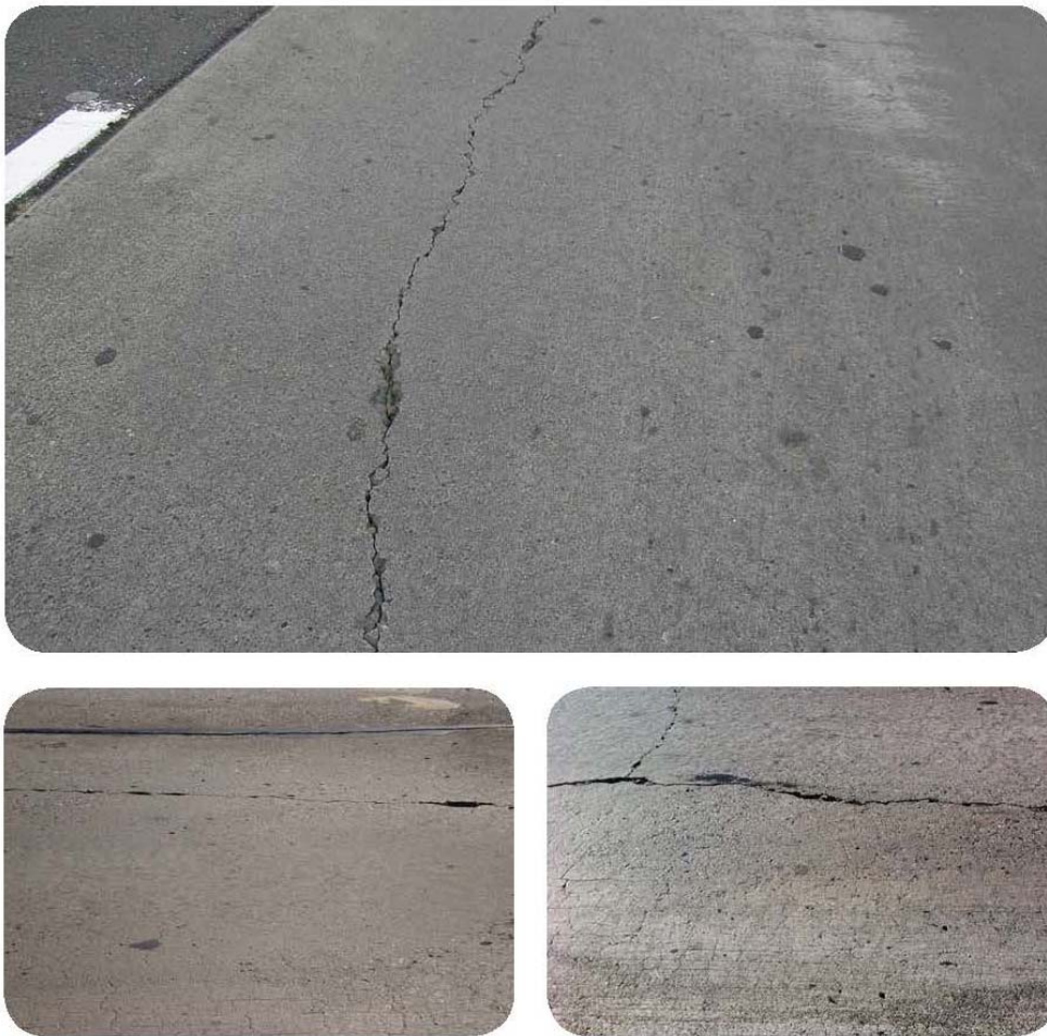
Figure 5-1. Examples of longitudinal cracks.
