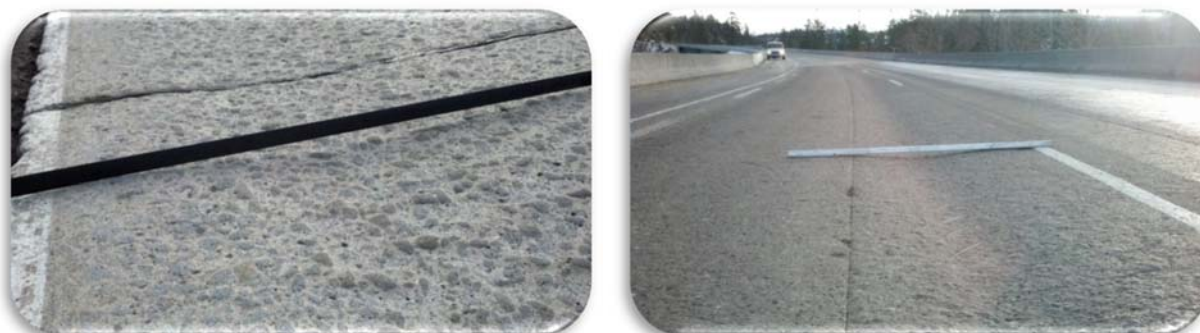
Figure 6-2. Examples of rutting in concrete.
