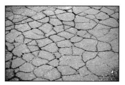
Figure 1: Chicken wire/alligator pattern cracking typical in fatigue cracking
