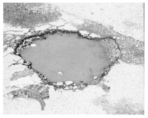
Figure 1. Pothole (photo courtesy The Asphalt Institute)
