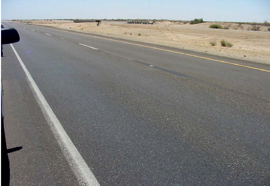
Figure 4. First pre-construction inspection with no signs of distress, July 2002 (Caltrans Maintenance – Ron Jones).
