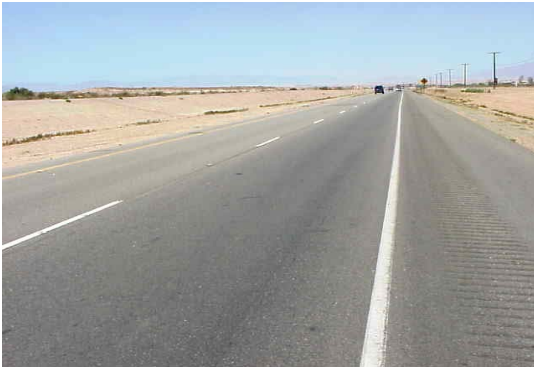
Figure 5. Second pre-construction inspection with no signs of distress, May 2003 (Caltrans Maintenance – Ron Jones).
