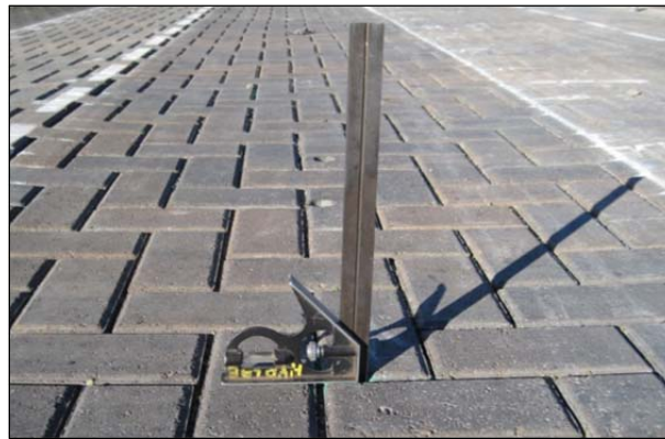
Figure 6.13: Jointing stone depth measurement.
