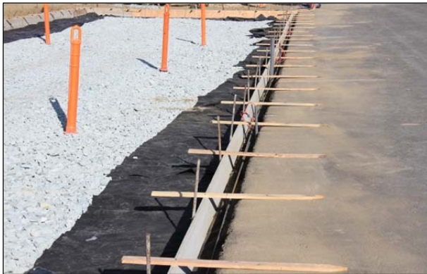
Figure 5.9: Formwork for curb.
