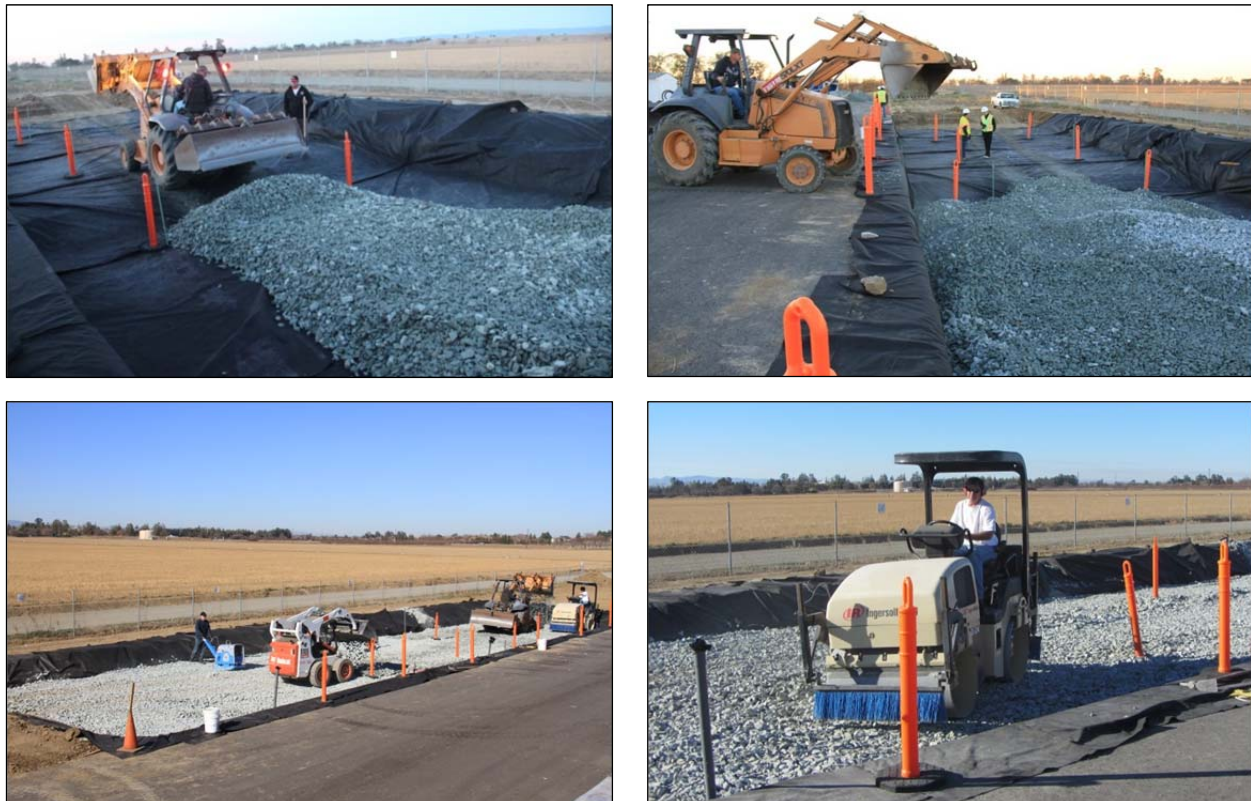
Figure 5.8: Placing and compacting the subbase.
