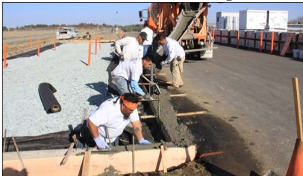
Figure 5.9: Formwork for curb.
