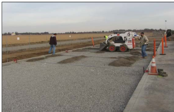
Figure 5.14: Bedding layer placement.
