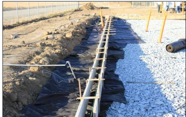
Figure 5.9: Formwork for curb.
