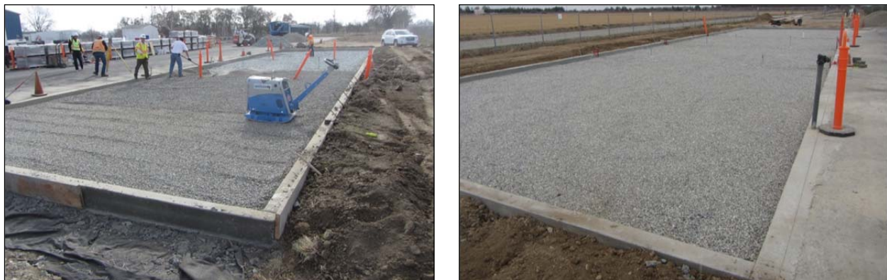
Figure 5.12: Base layer placement.
