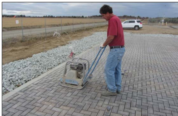
Figure 5.15: Paver placement and compaction.
