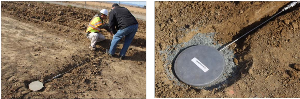
Figure 6.10: Pressure cell installation in the subgrade.
