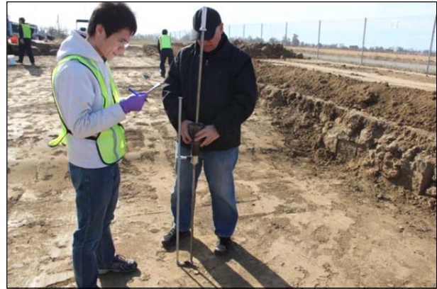
Figure 5.6: Dynamic cone penetrometer measurements.
