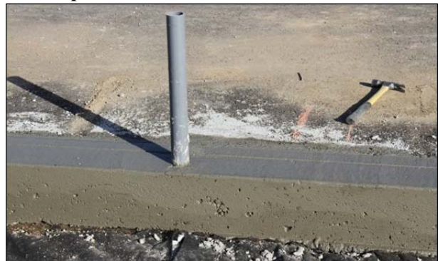
Figure 5.11: Completed curb after removal of formwork (pipes are for instrument wiring).
