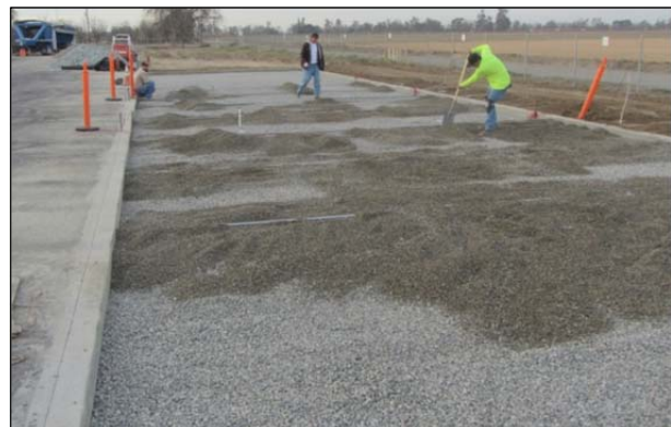
Figure 5.14: Bedding layer placement.
