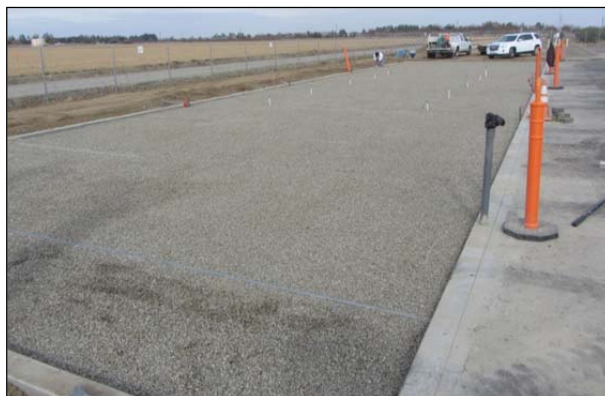
Figure 5.13: Bedding layer placement.
