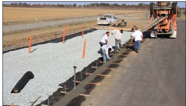
Figure 5.9: Formwork for curb.
