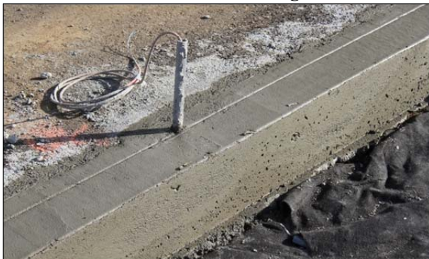
Figure 5.11: Completed curb after removal of formwork (pipes are for instrument wiring).
