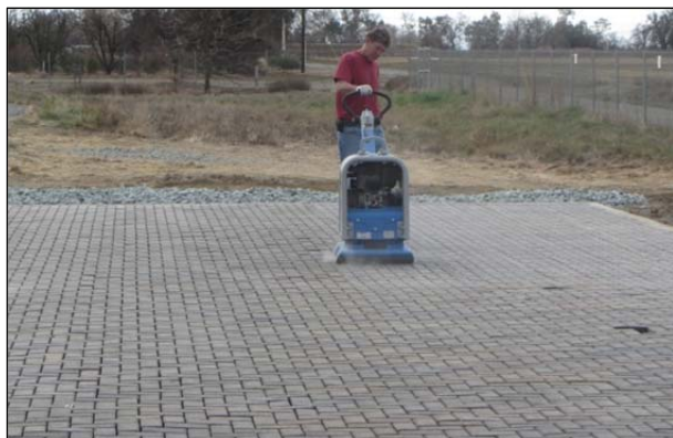
Figure 5.15: Paver placement and compaction.
