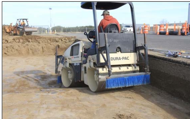
Figure 5.2: Subgrade compaction.
