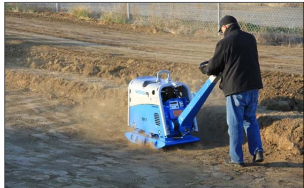
Figure 5.2: Subgrade compaction.
