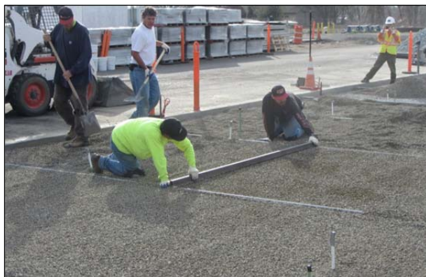
Figure 5.13: Bedding layer placement.
